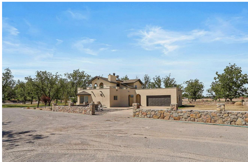
EXISTING SINGLE FAMILY RESIDENCE
