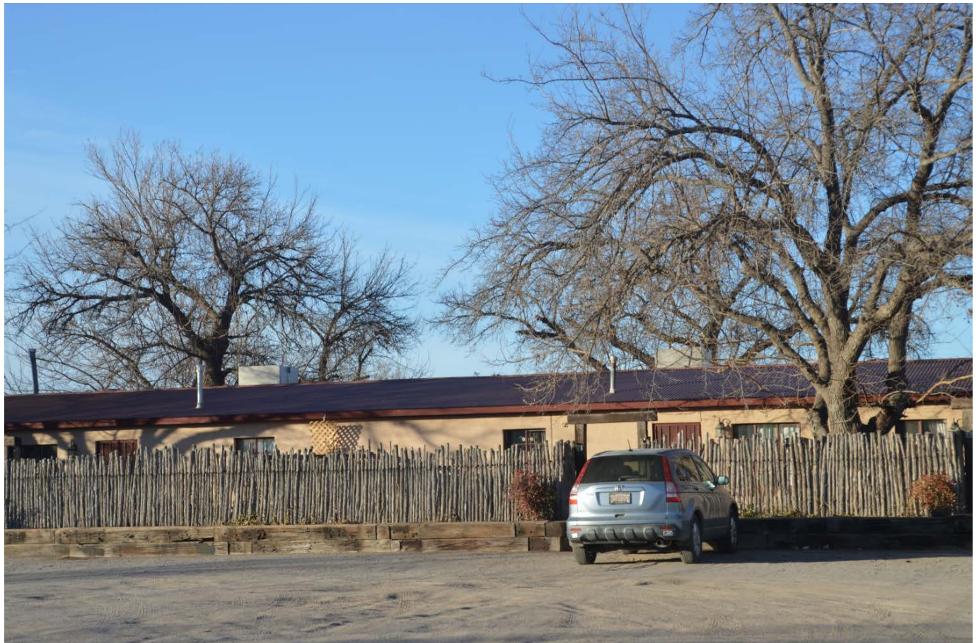
PHOTO OF THE APARTMENTS TO THE EAST SHOWING THE PITCHED ROOF
