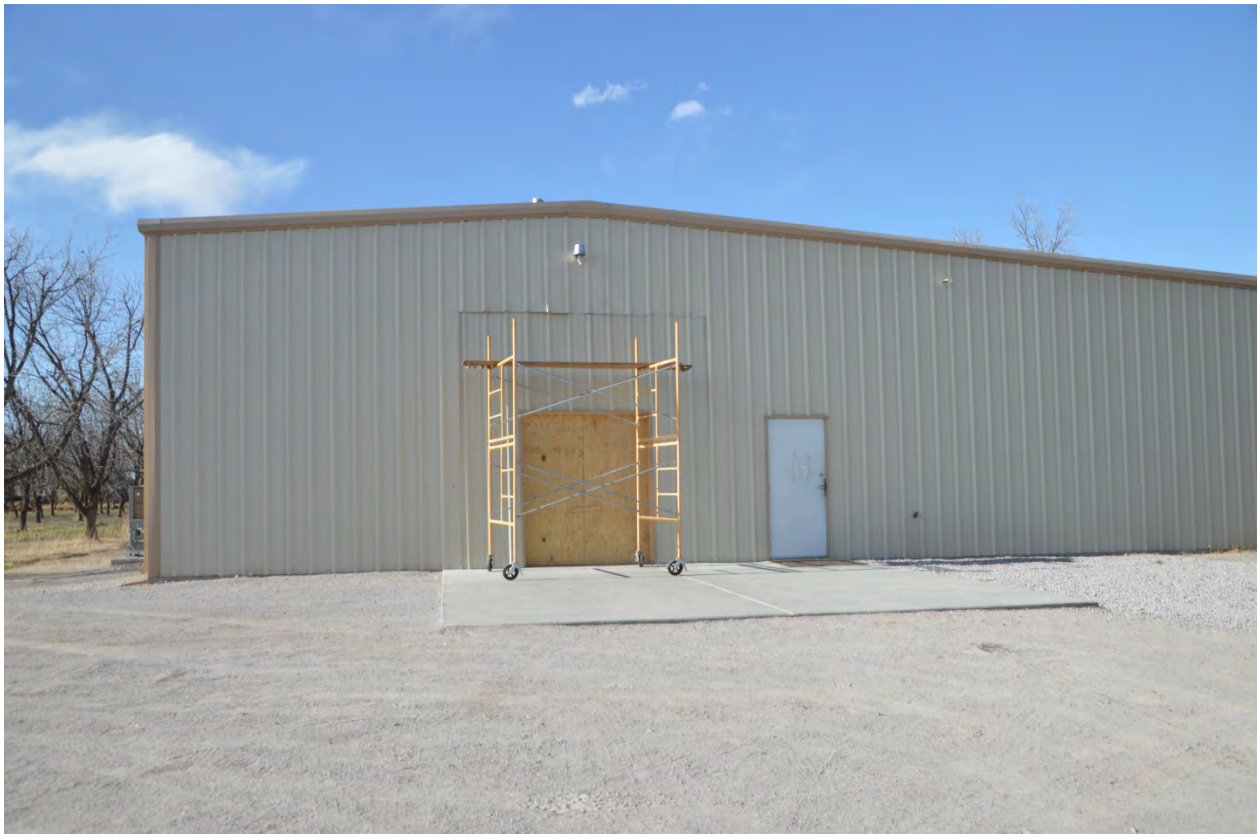
VIEW OF METAL BUILDING FROM UNIVERSITY AVENUE
