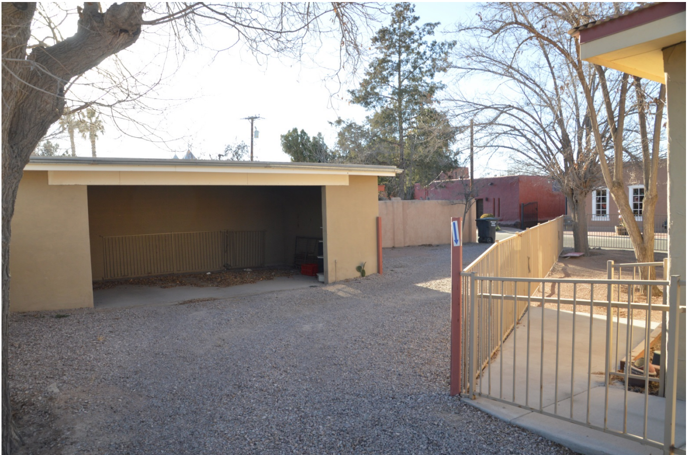
PHOTO OF THE GARAGE AT THE REAR OF THE STRUCTURE
