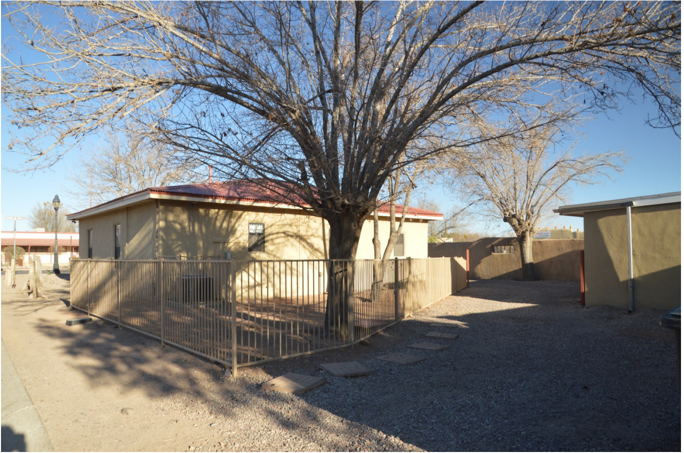
PHOTO OF THE REAR OF THE STRUCTURE FROM CALLE DE SANTIAGO
