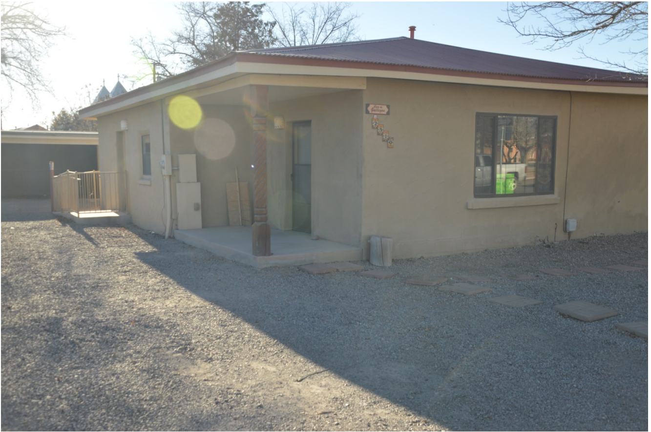
PHOTO OF THE FRONT ENTRANCE TO THE STRUCTURE
