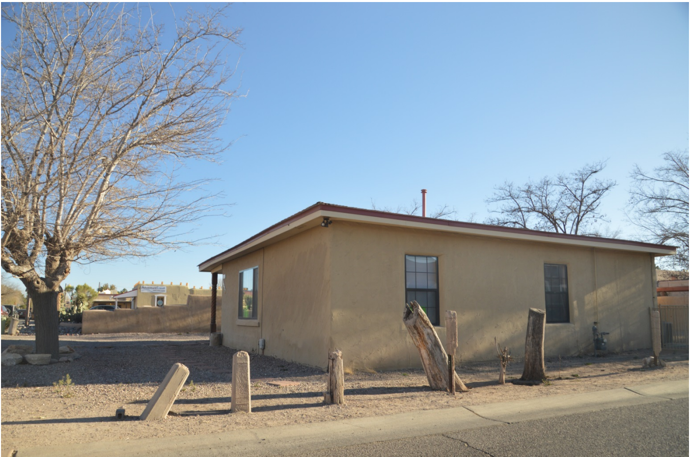
PHOTO OF THE STRUCTURE FROM CALLE DE SANTIAGO
