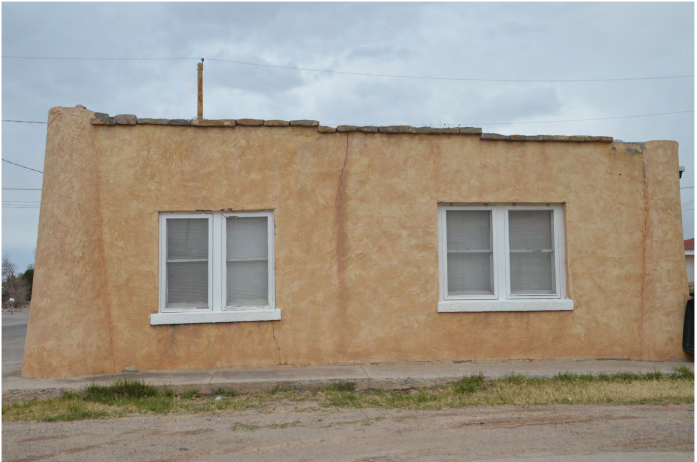
PHOTO OF DWELLING FROM CALLE DE SAN ALBINO
