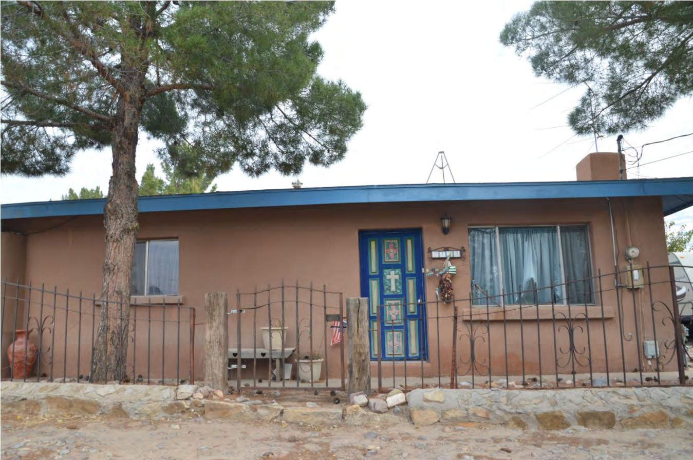
PHOTO FROM CALLE DE SAN ALBINO OF FRONT OF STRUCTURE TO BE DEMOLISHED
