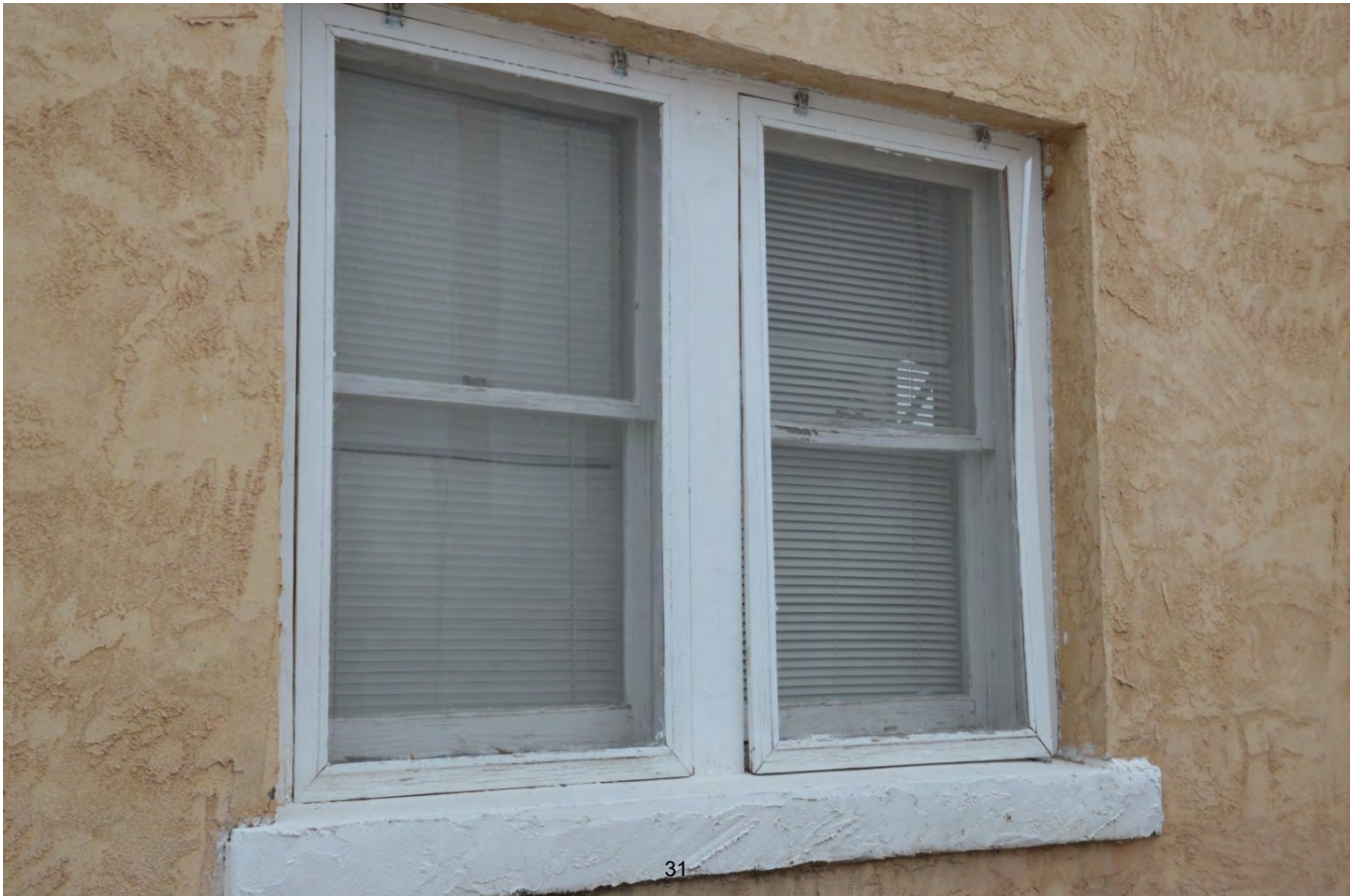
PHOTOS OF WINDOWS TO BE REPLACED
