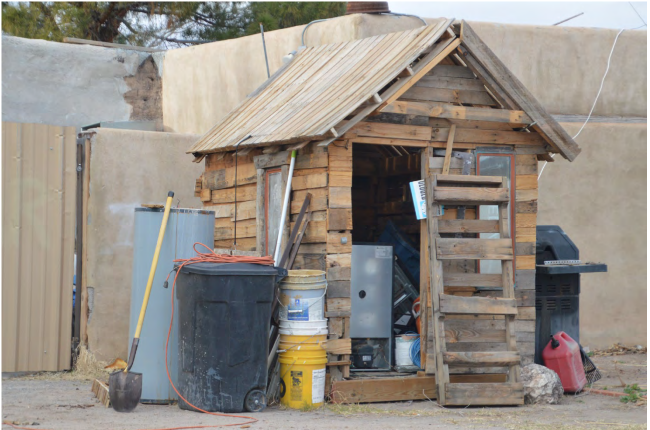
PHOTO OF SHED
