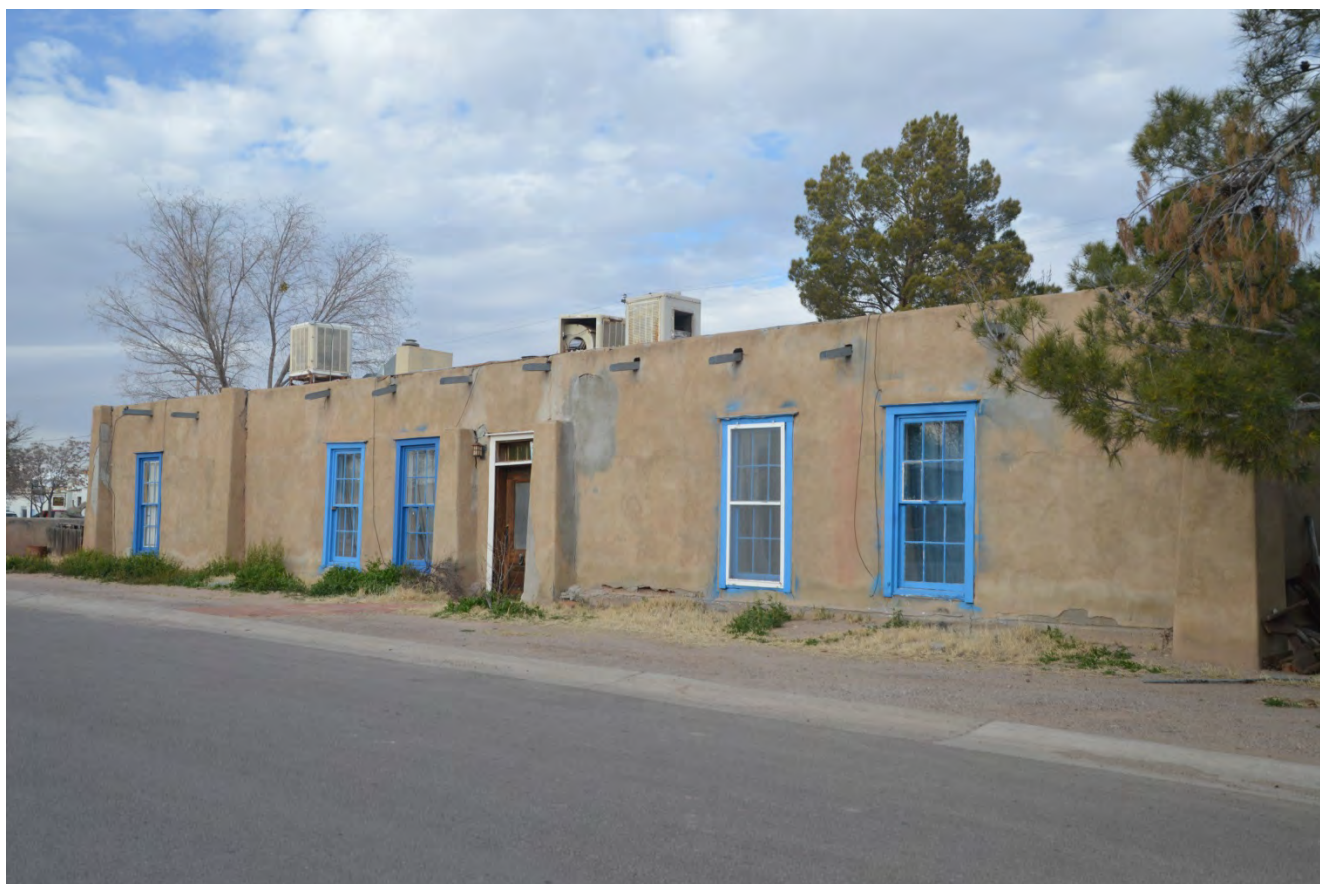
PHOTO OF DWELLING FROM CALLE PRINCIPAL SHOWING WINDOWS AND TRIM, ALONG WITH ORIGINAL DWELLING COLOR
