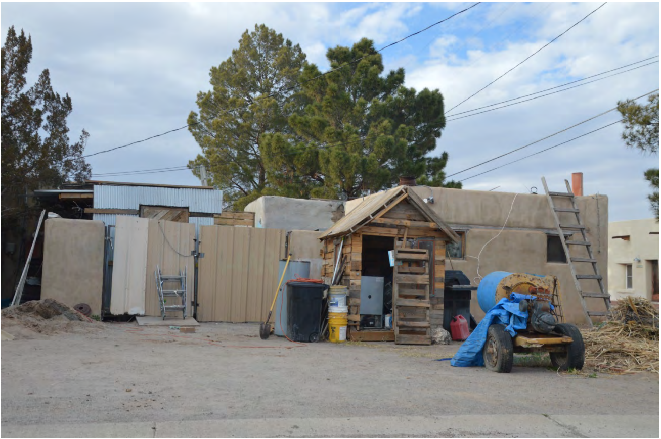
PHOTO OF SOUTH SIDE OF PROPERTY FROM CALLE DE COLON SHOWING SHED AND AREA TO BE FENCED
