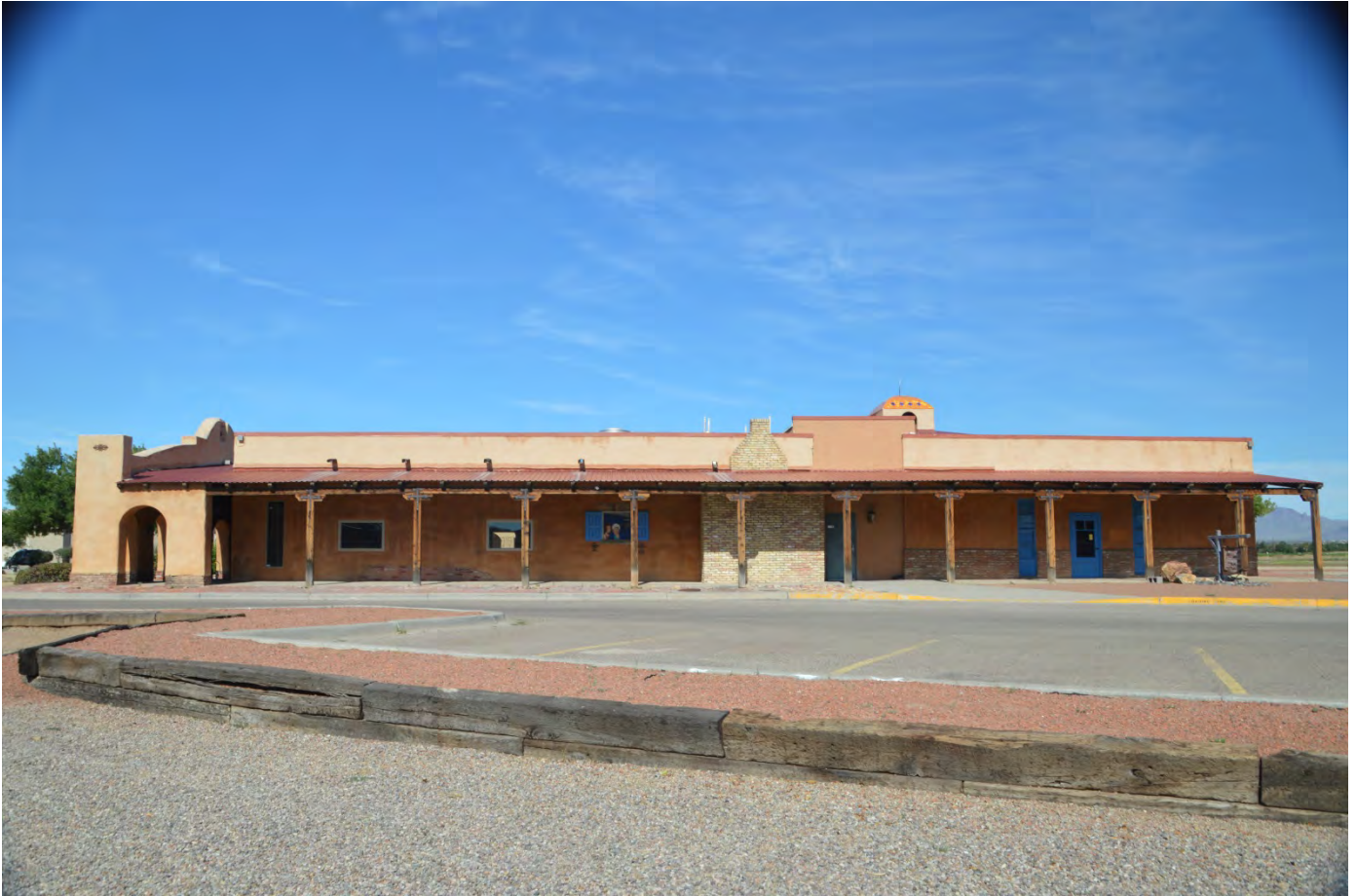
VIEW OF THE STRUCTURE FROM THE WEST
