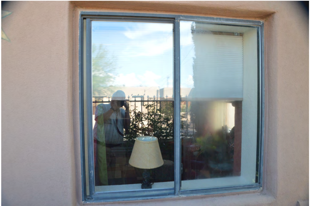
VIEW OF WINDOW AT FRONT OF DWELLING
