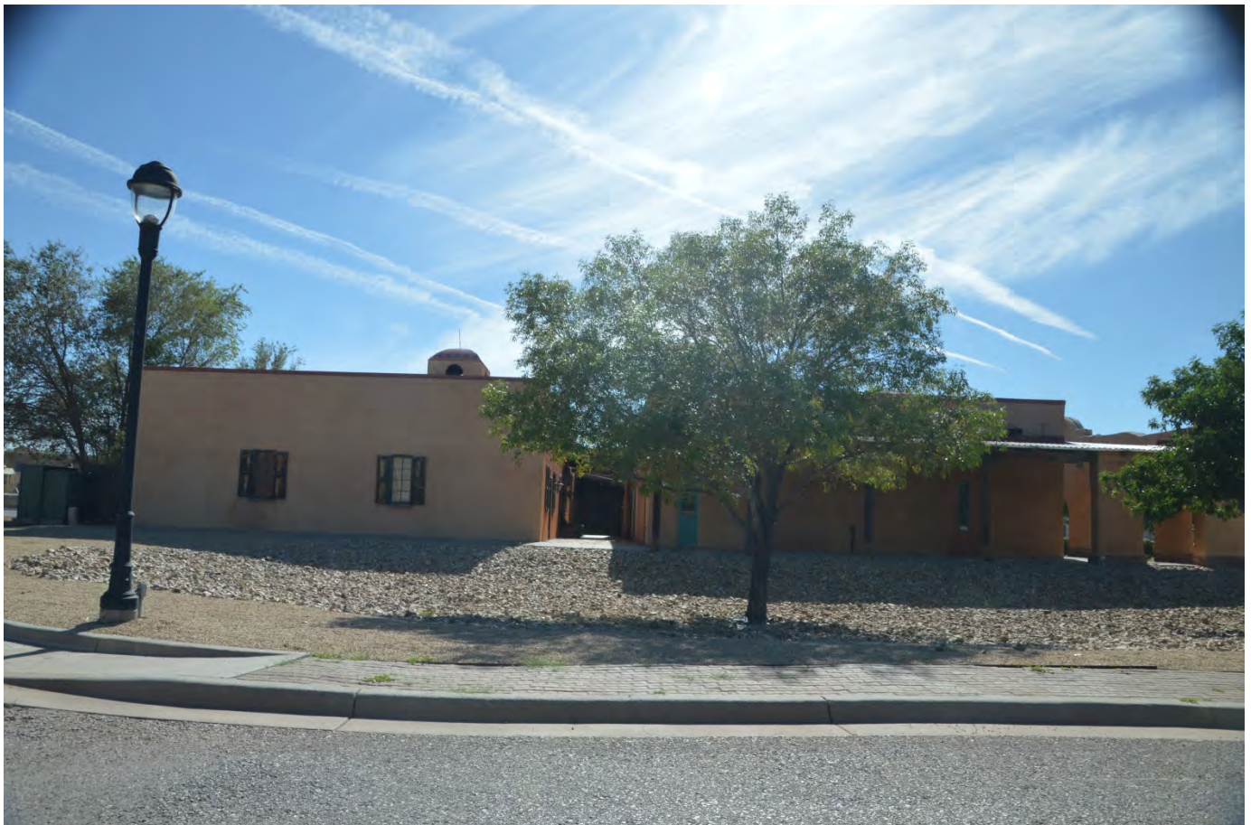
VIEW OF THE STRUCTURE FROM THE EAST
