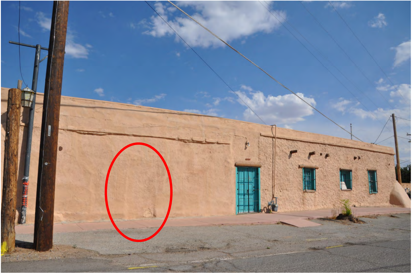
PHOTO OF SUBJECT STRUCTURE FROM CALLE DE PARIAN (STREET SIDE)
