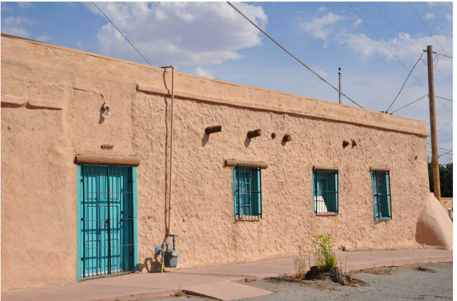
PHOTOS OF SUBJECT STRUCTURE FROM CALLE DE PARIAN (STREET SIDE)
