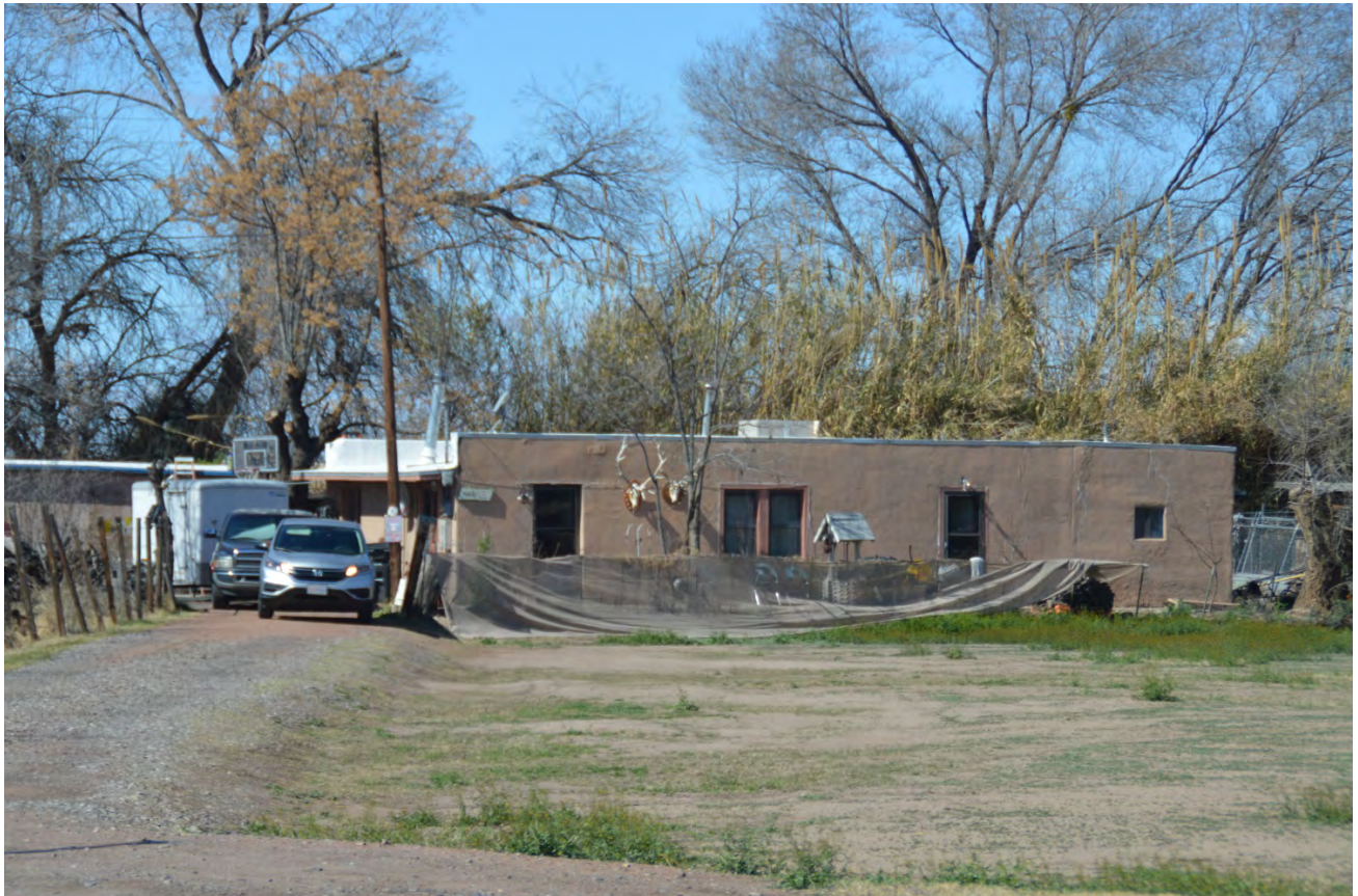
PHOTO OF THE DWELLING AT 2170 CALLE DEL NORTE
