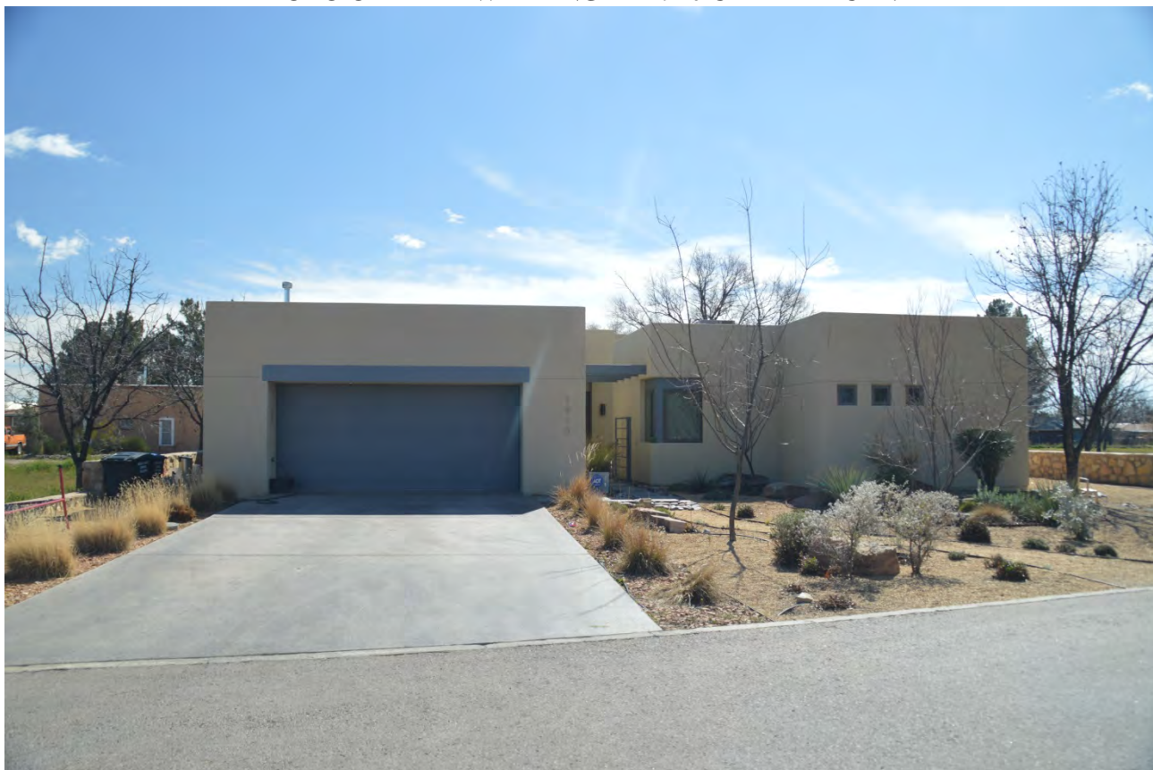
PHOTO OF THE DWELLING AT 1910 CALLE PACANA
