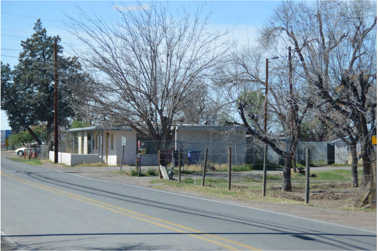
PHOTO OF THE DWELLING AT 2188 CALLE DEL NORTE
