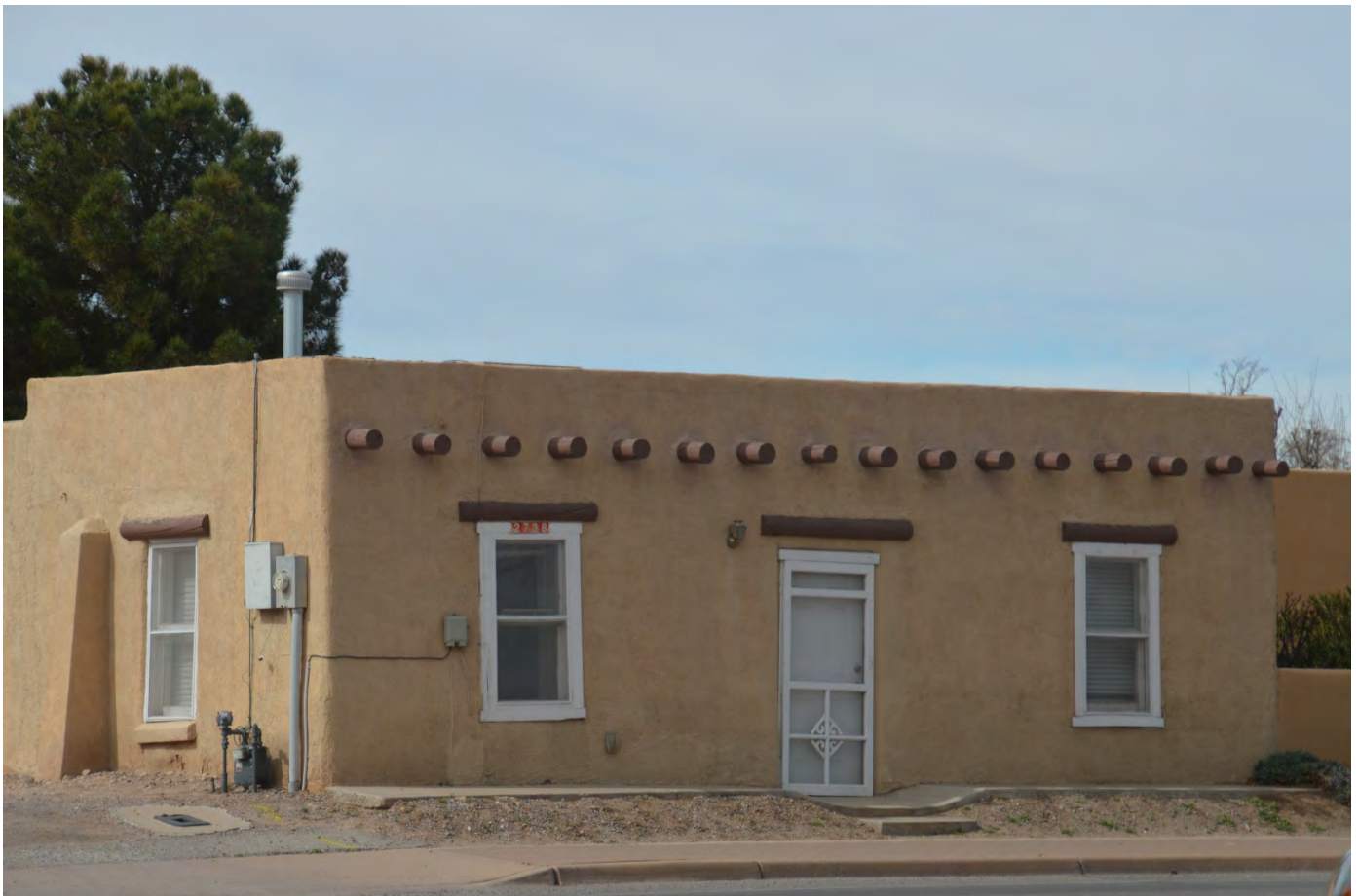
PHOTO OF NEARBY RESIDENTIAL RENTAL UNIT
