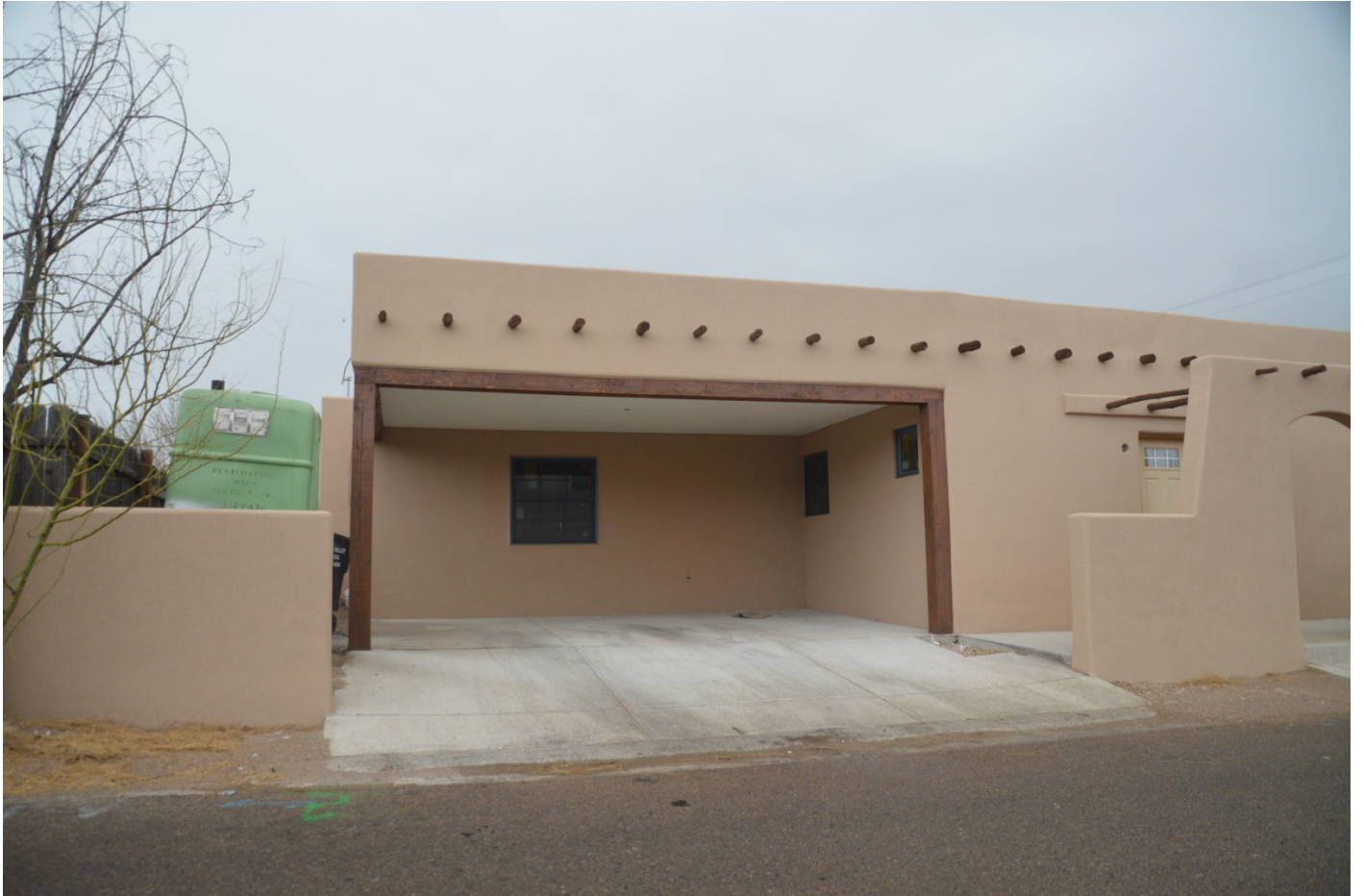
PHOTO OF PROPERTY FROM CALLE DE MEDANOS SHOWING WEST DRIVEWAY
