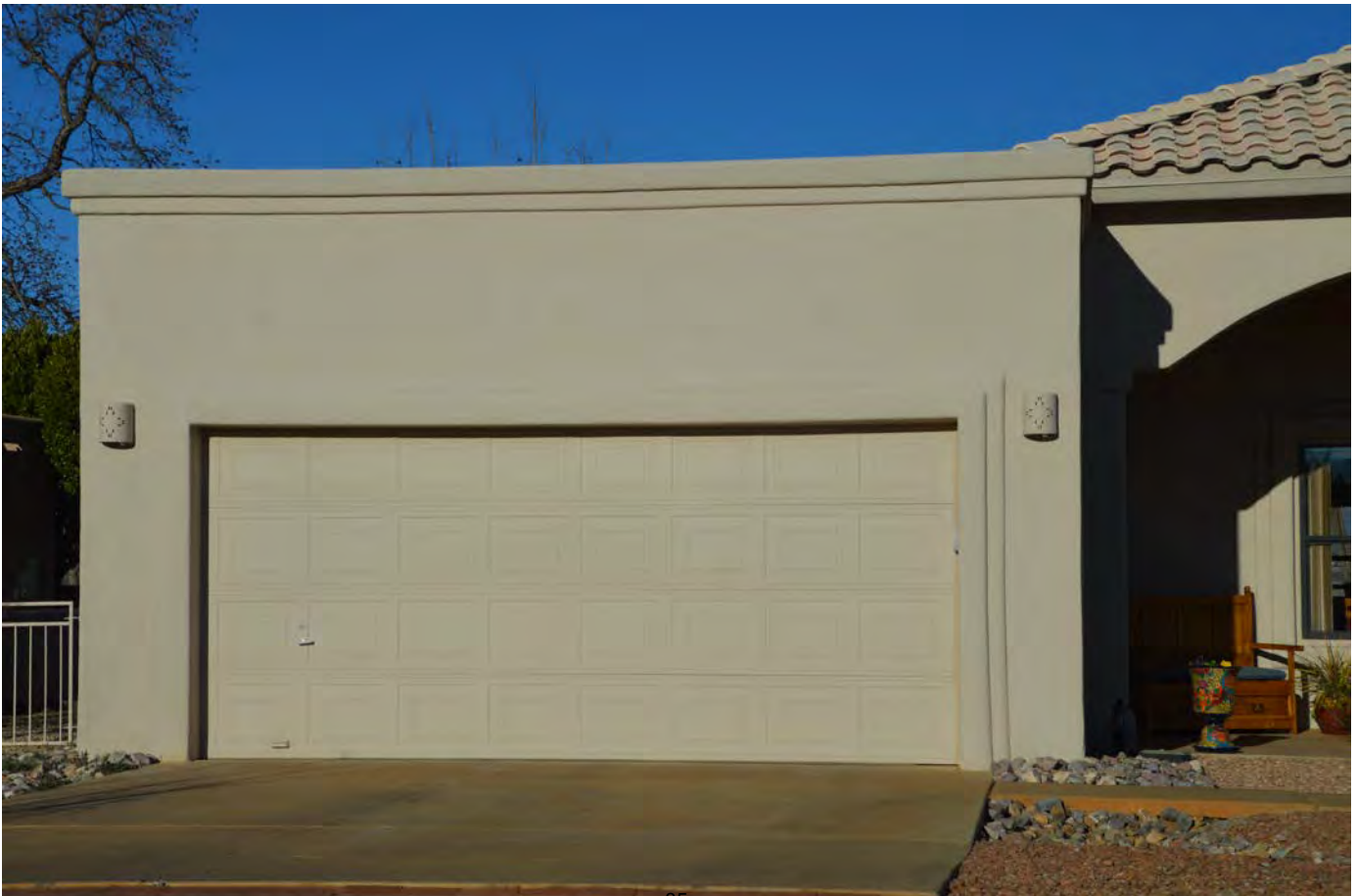
CLOSE-UP OF GARAGE FROM BOLDT STREET SHOWING TRIM
