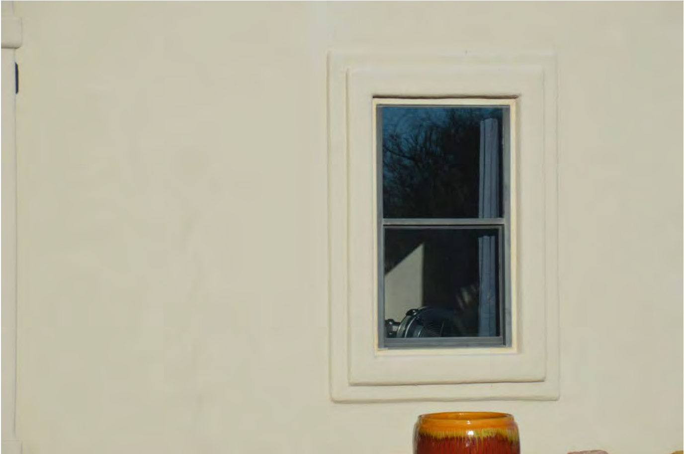
CLOSE-UP OF WINDOW FROM BOLDT STREET SHOWING TRIM
