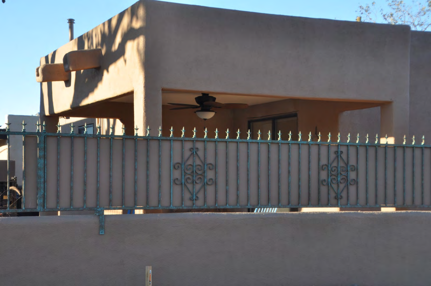
VIEW OF DWELLING AND PATIO FROM CALLE DE MEDANOS
