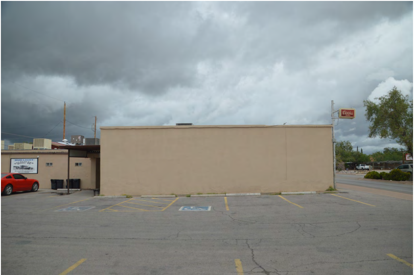
PHOTO OF EXTERIOR WALL TO BE PAINTED WITH MURAL
