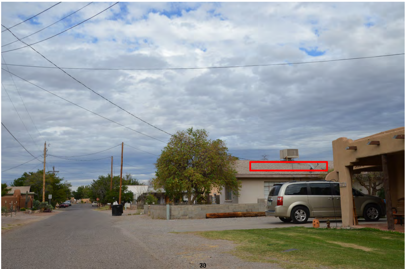
PHOTO OF DWELLING FROM CALLE DE SANTIAGO, FACING EAST
