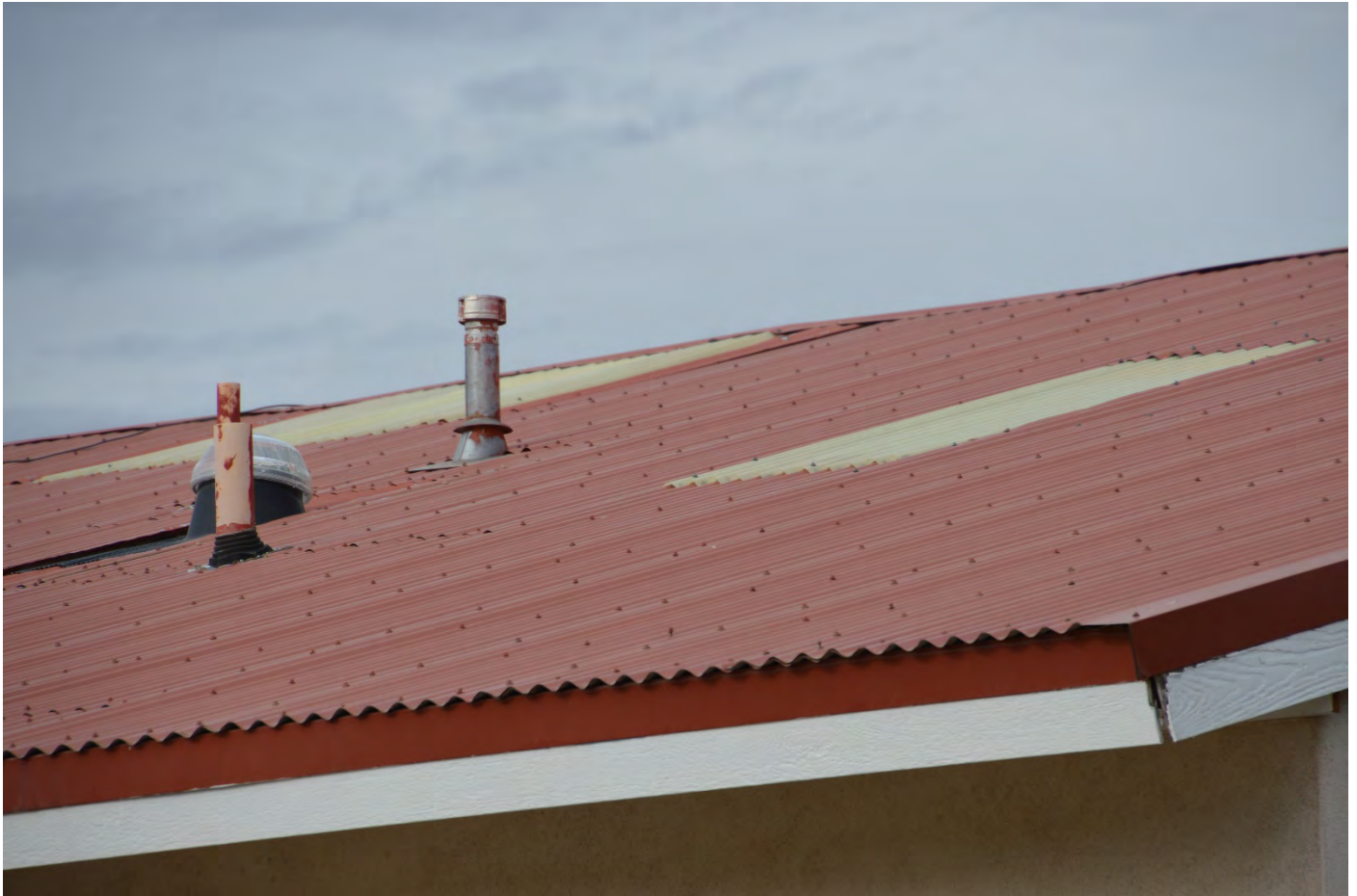
PHOTO OF THE DWELLING SHOWING THE EXISTING ROOF
