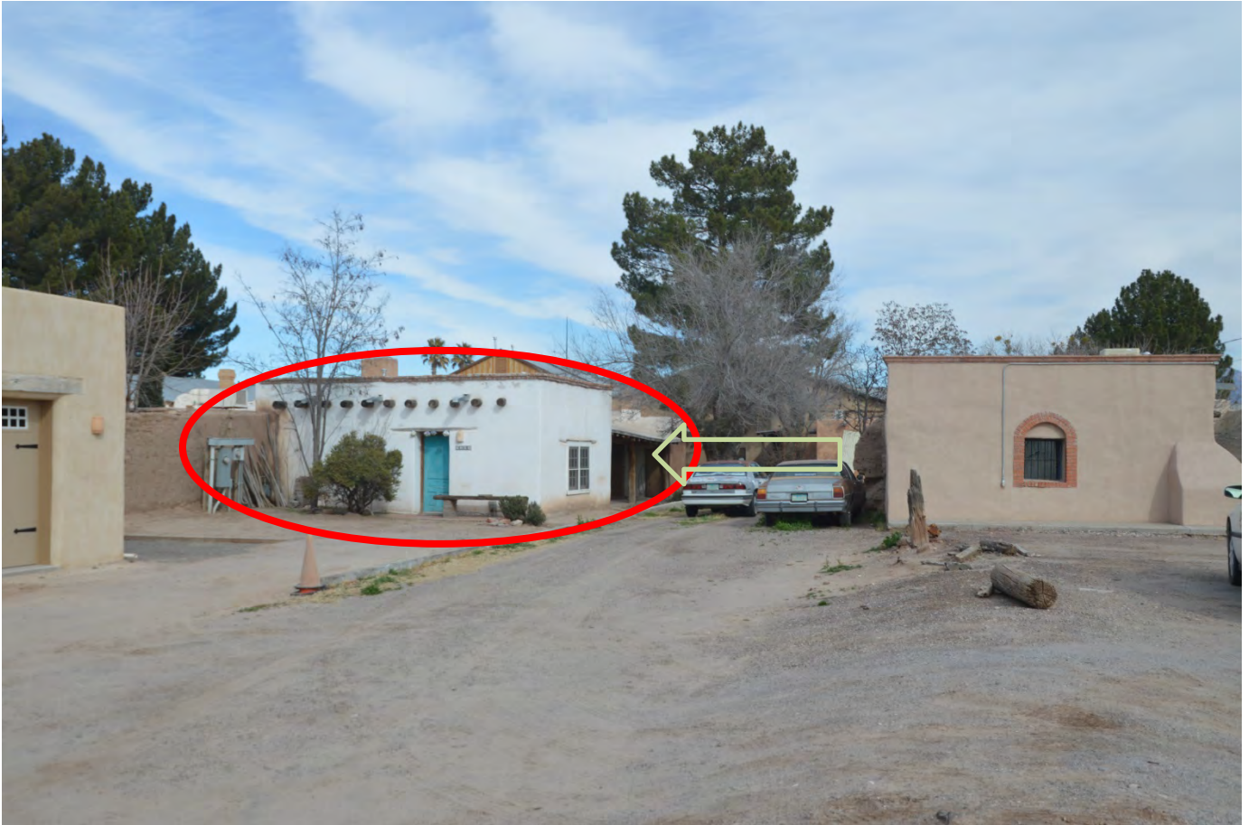
PHOTO OF DWELLING FROM CALLE DE ARROYO (ARROW POINTS TO WINDOW UNDER PORCH)
