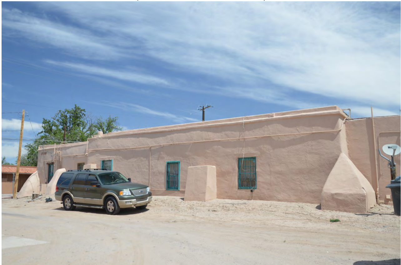
PHOTO OF THE PROPERTY FROM THE NORTH (FROM CALLE DE PARIAN)
