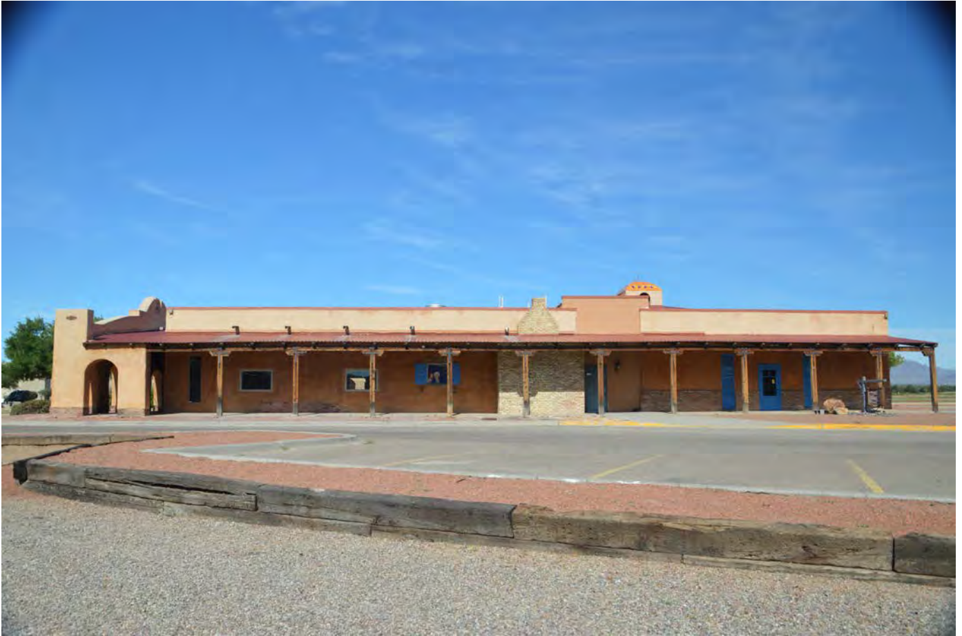
VIEW OF THE STRUCTURE FROM THE WEST
