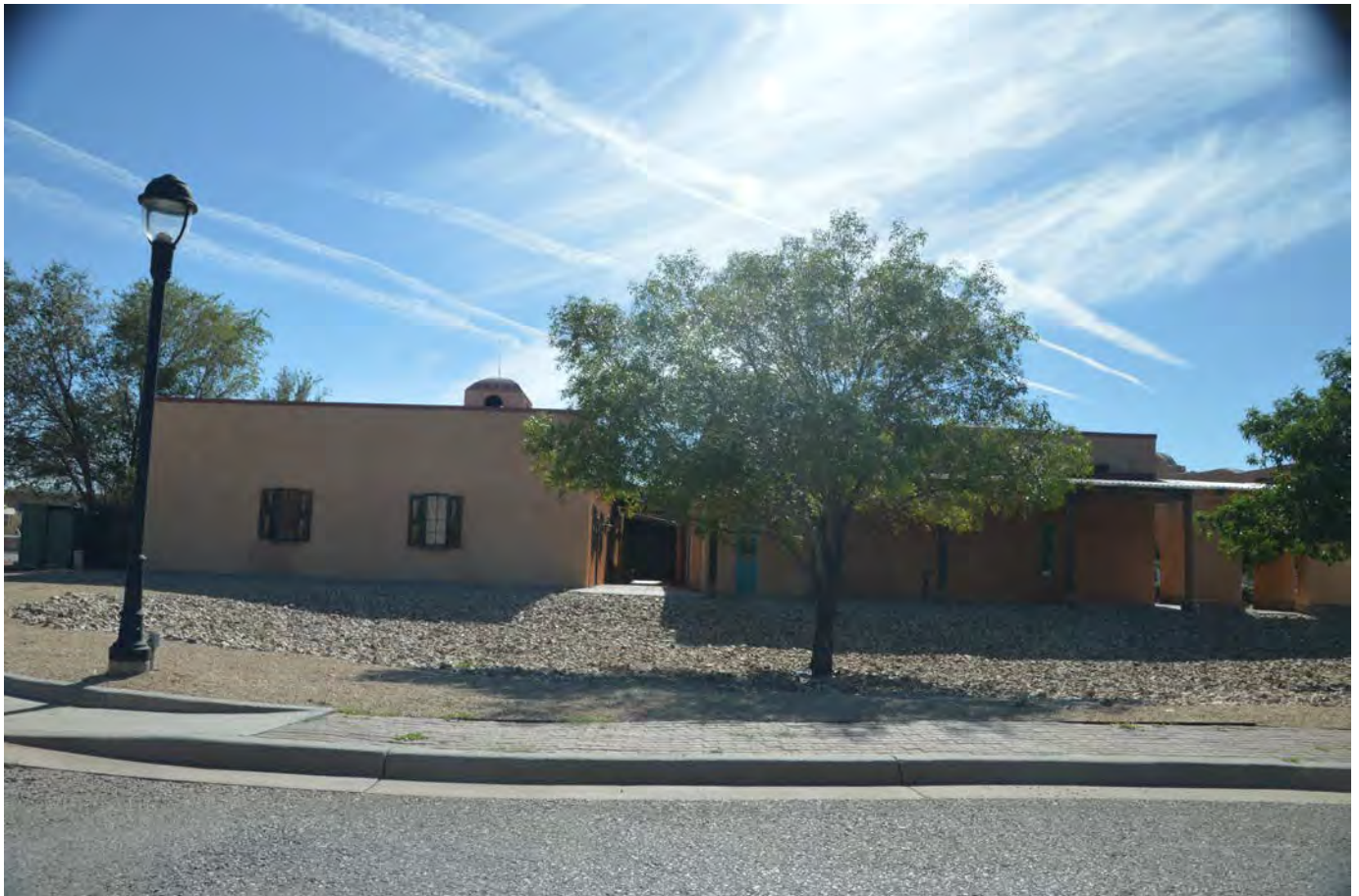
VIEW OF THE STRUCTURE FROM THE EAST
