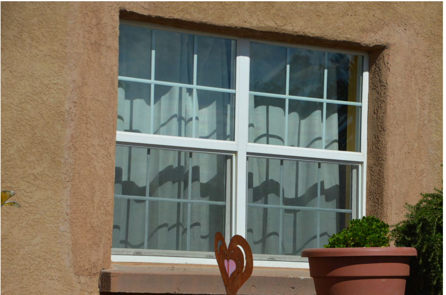
VIEW OF WINDOW AT 2149 CALLE DE GUADALUPE (EXAMPLE O REPLACEMENT STYLE)
