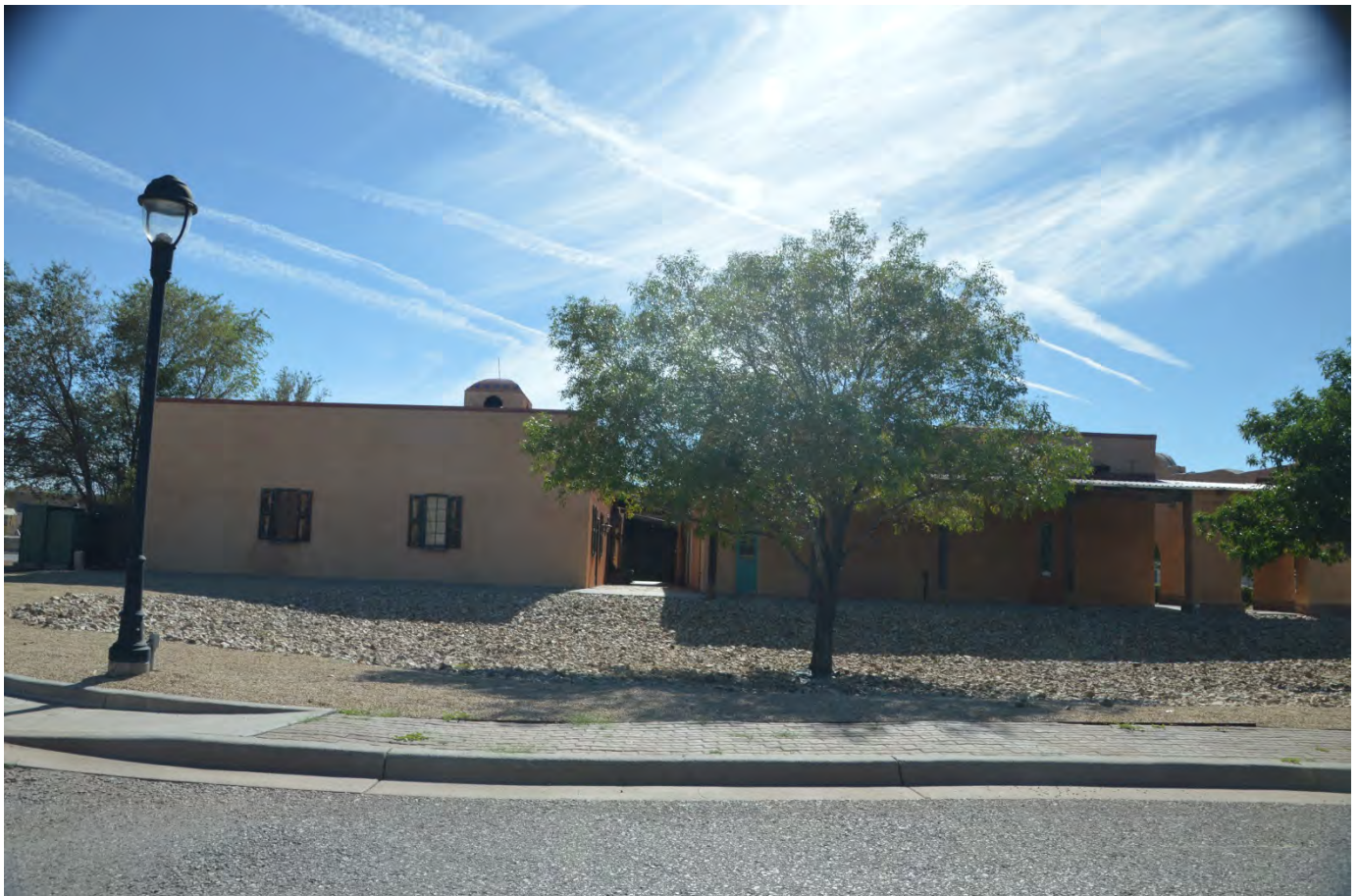
VIEW OF THE STRUCTURE FROM THE EAST
