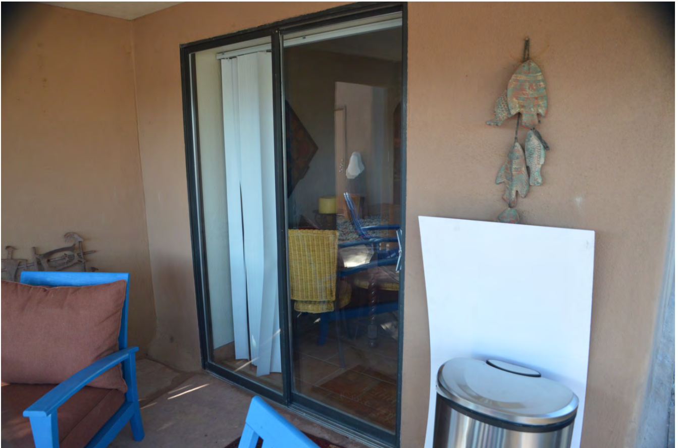
VIEW OF WINDOWS ON REAR SIDE OF DWELLING
