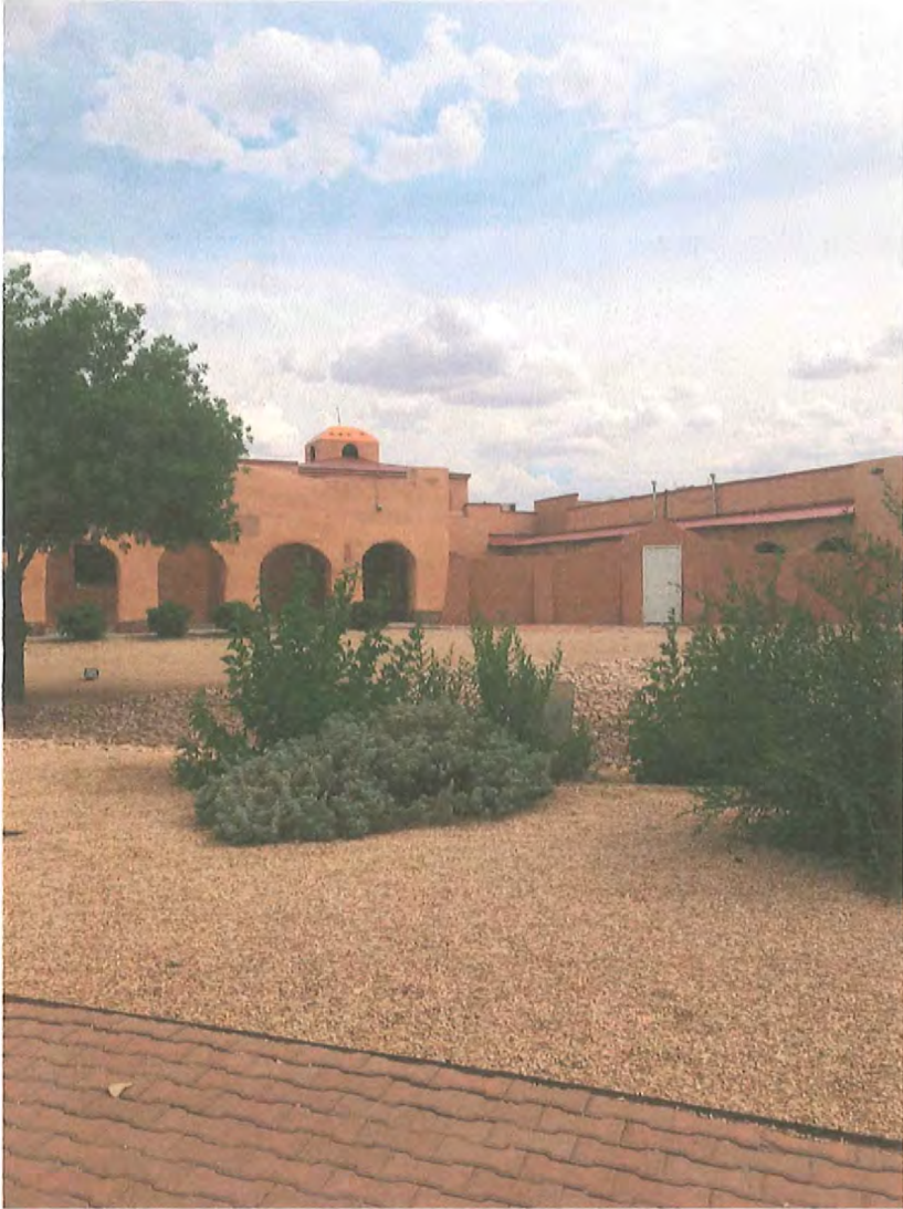
Remove the solid courtyard wall and replace it with a new landscape design per supplied plans.
