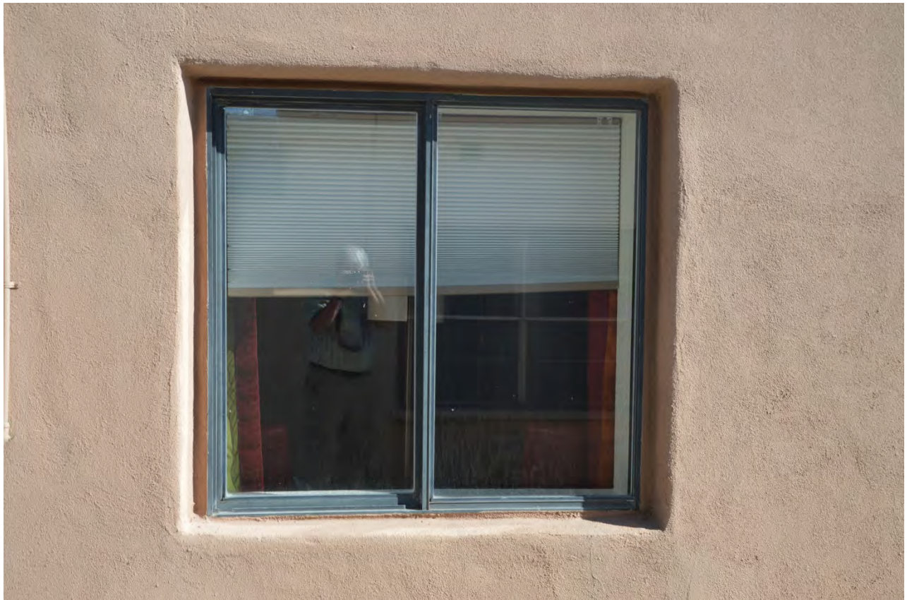
VIEW OF WINDOW ON NORTH SIDE OF DWELLING
