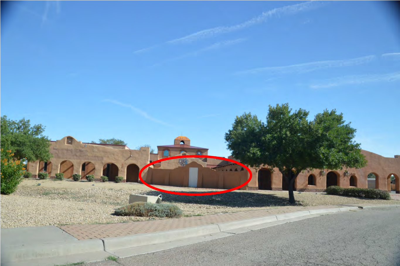
VIEW OF THE STRUCTURE FROM THE FRONT (NORTH)
