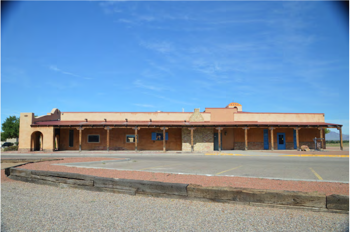
VIEW OF THE STRUCTURE FROM THE WEST
