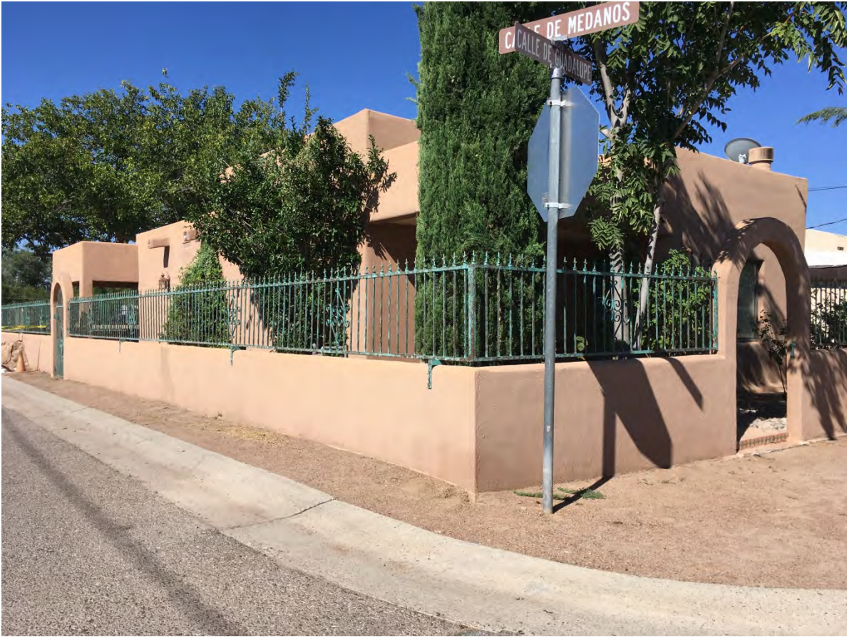
VIEW OF FRONT OF PROPERTY FROM CALLE DE MEDANOS
