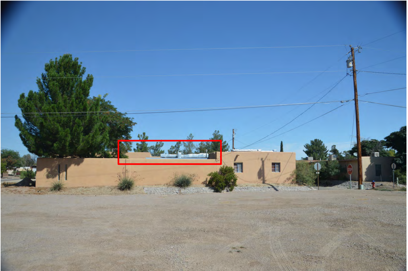
PHOTOS OF DWELLING LOOKING NORTH FROM CALLE DE SANTA ANA SHOWING PART OF WALL TO BE AFFECTED BY ADDITION
