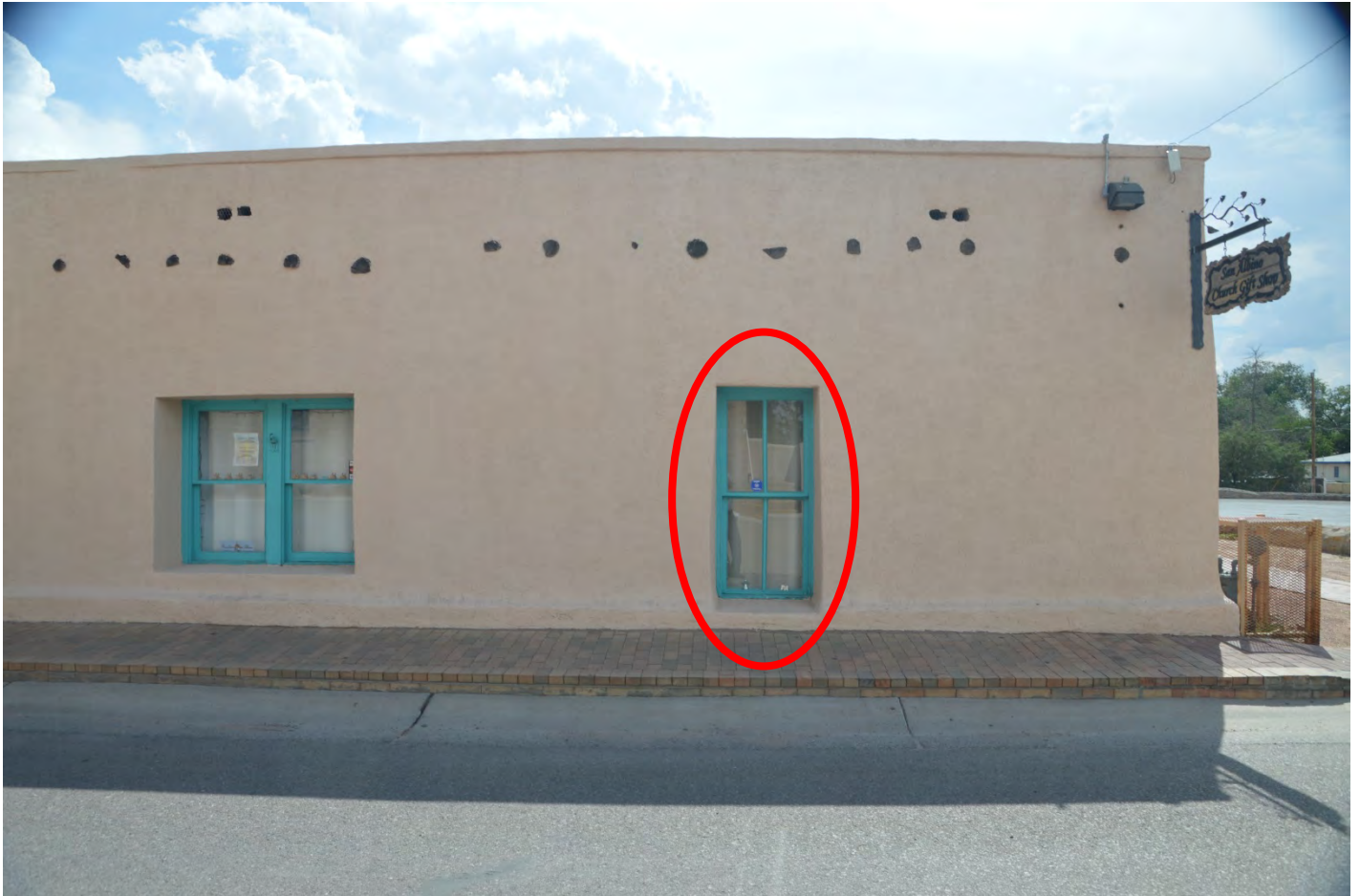
PHOTOS OF WINDOW TO BE REPLACED BY NEW DOOR
