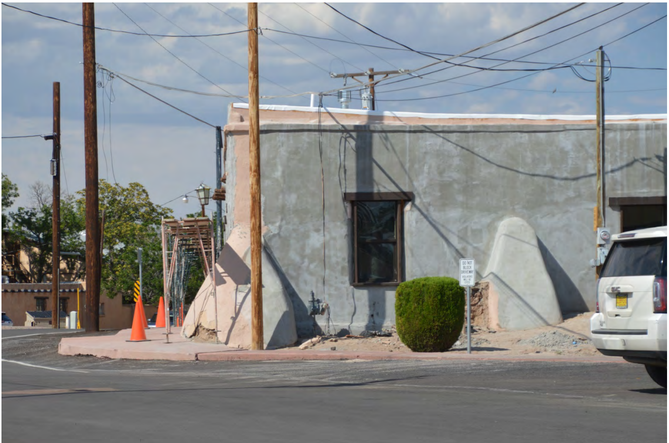
PHOTO OF DWELLING AND SIDEWALK FROM CALLE DE PARIAN
