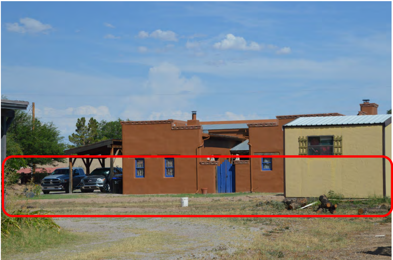
REAR SIDE OF THE PROPERTY SHOWING THE PROPOSED WALL LOCATION FROM THE NEIGHBORING PROPERTY
