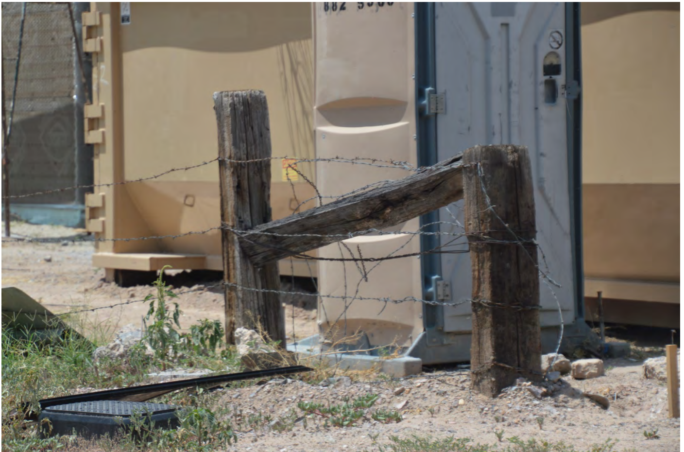
VIEW OF PART OF WIRE FENCE ADJACENT TO CALLE DE SEGUNDA
