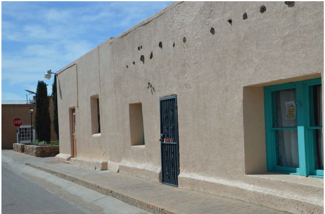
PHOTO OF WALL SHOWING OTHER DOORS
