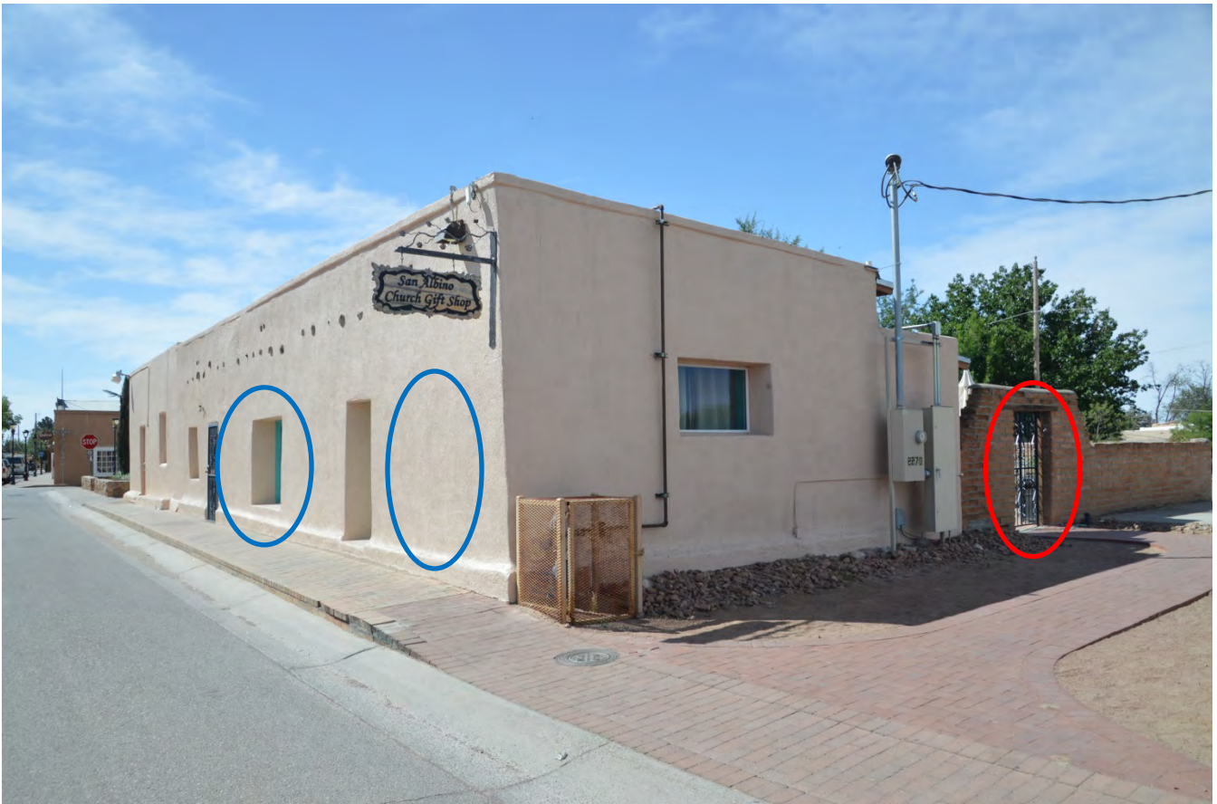
PHOTO OF FRONT OF STORE SHOWING CURRENT ENTRANCE AND ALTERATIVE ENTRANCES
