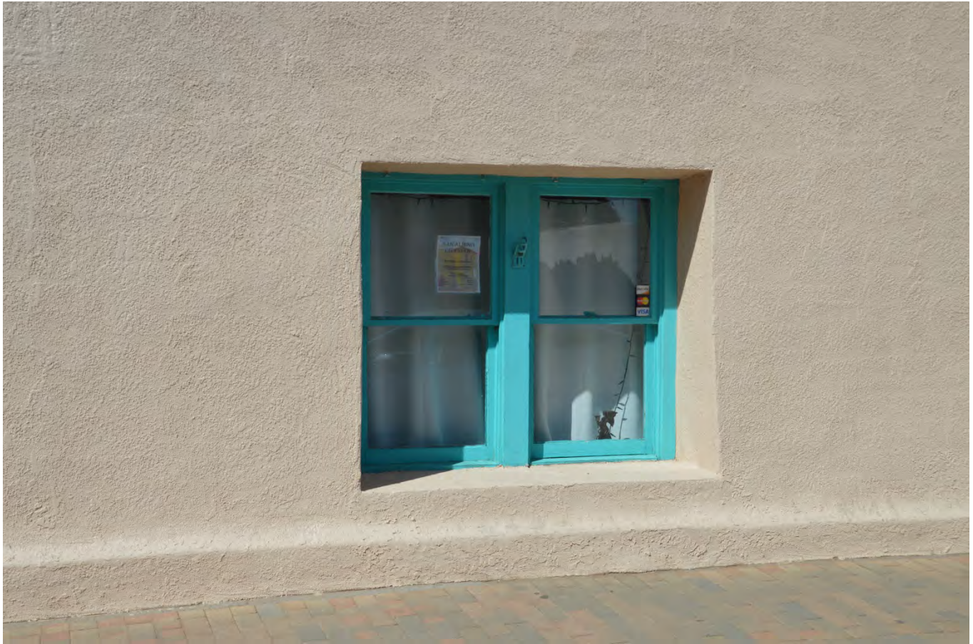
PHOTO OF WINDOW TO BE REPLACED BY NEW DOOR
