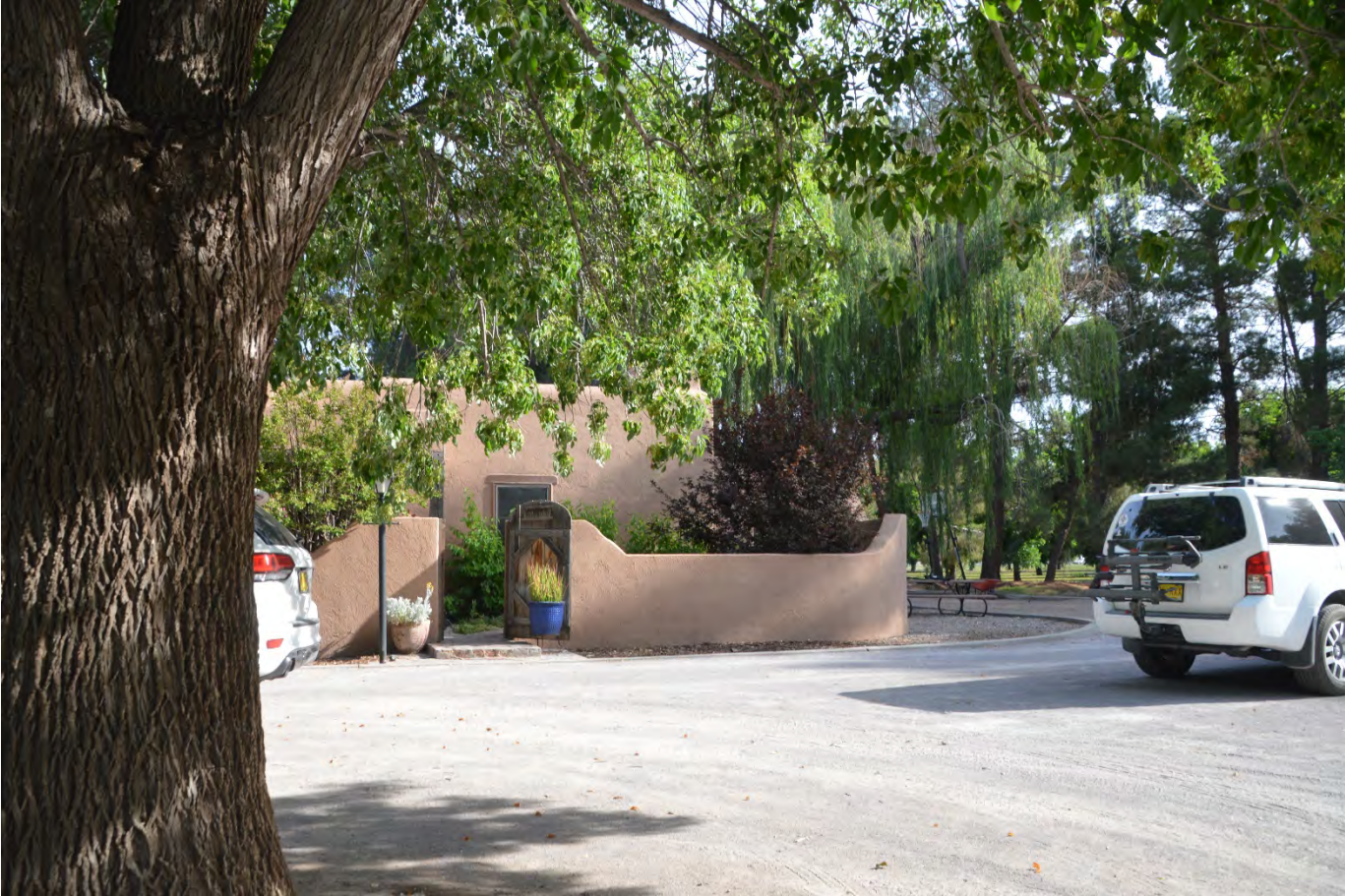
NORTH SIDE OF THE DWELLING SHOWING EXISTING PARKING FOR VEHICLES
