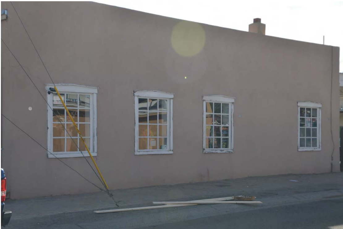
PHOTO OF SUBJECT STRUCTURE FROM CALLE DE PRINCIPAL
