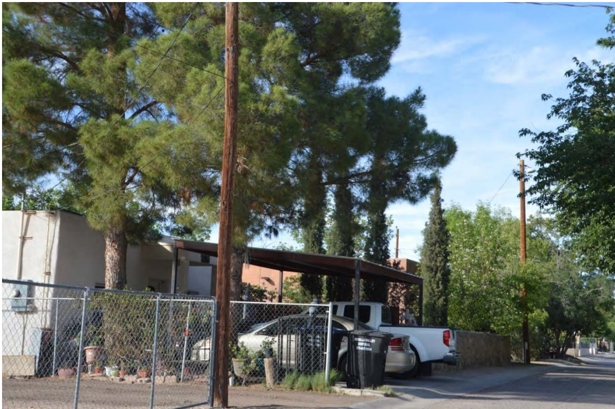
VIEW OF THE CARPORT FROM CALLE DE CURA
