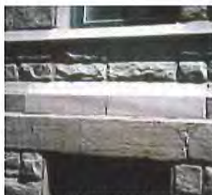
Replacement stones tooled to
