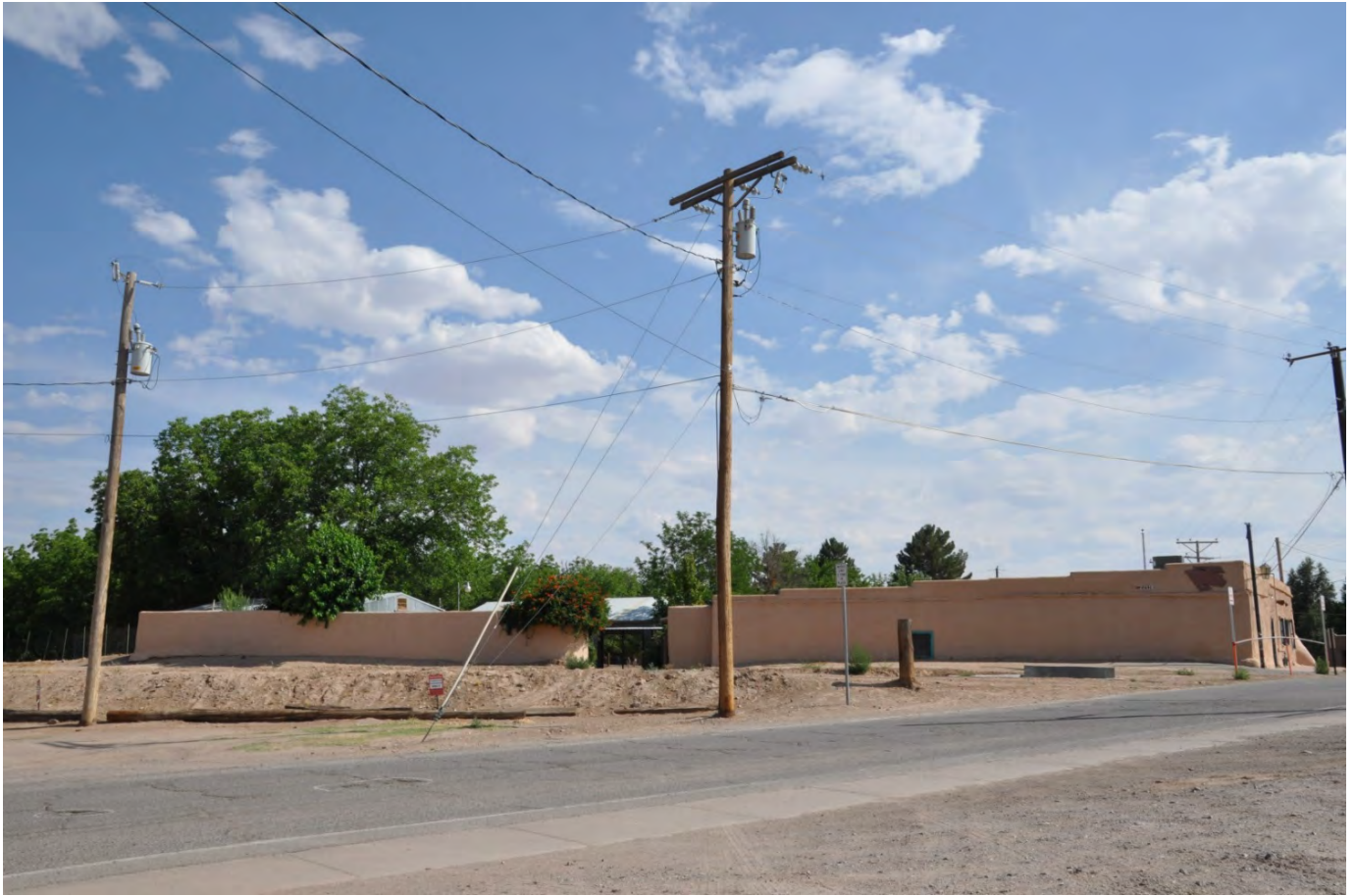
VIEW OF EAST SIDE OF PROPERTY
