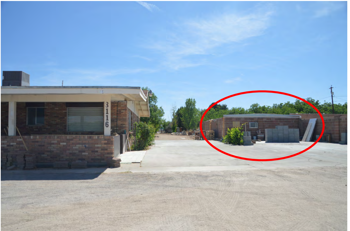
PHOTO SHOWING THE EAST SIDE OF THE MAIN DWELLING AND STORAGE STRUCTURE
