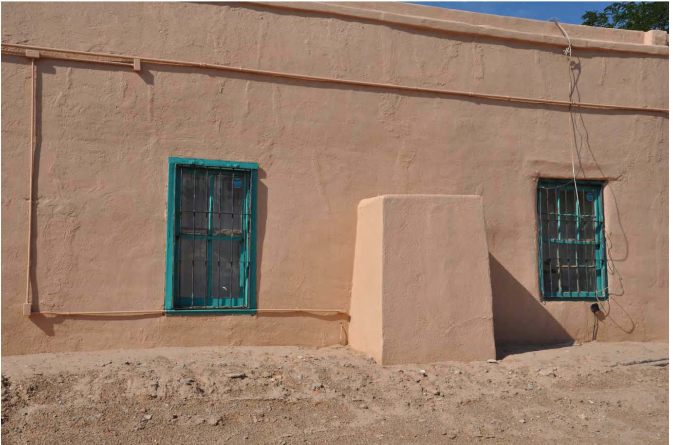
VIEW OF WINDOWS ON SOUTH SIDE OF STRUCTURE
