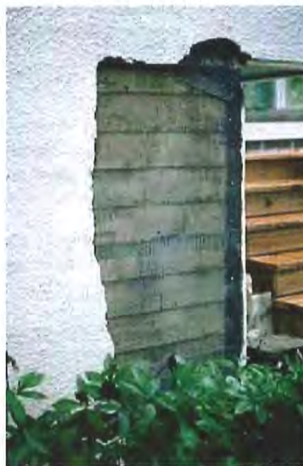
Preparation for stucco repair.
