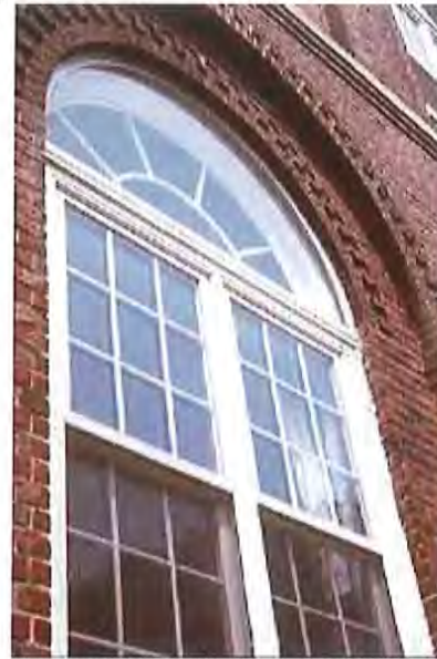
Newly painted double-hung wood windows.
