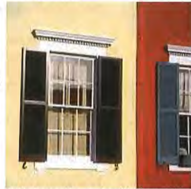
Delicate muntins and multi-pane sash on early 19th c. row houses.
