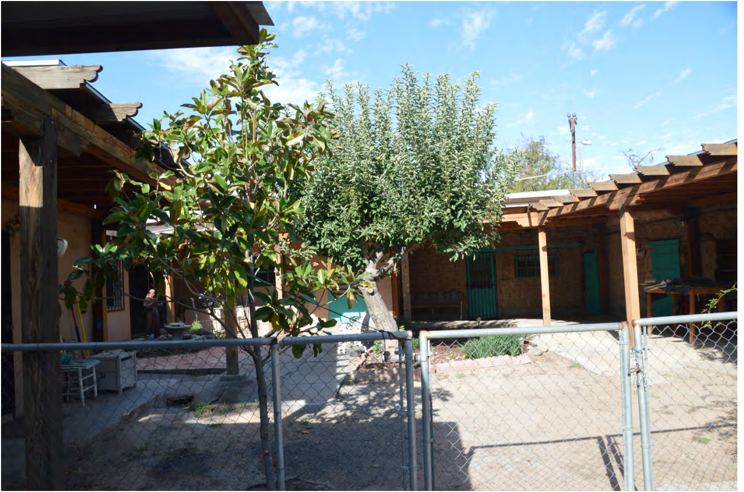
PHOTOS OF THE COURTYARD AT THE REAR OF THE DWELLING (SOUTH SIDE)
