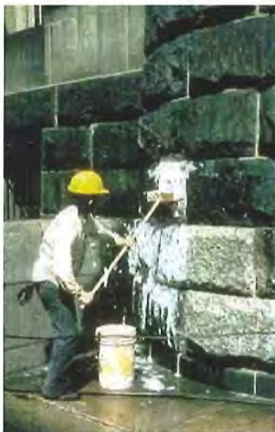
Chemical cleaning to remove dirt from granite.
