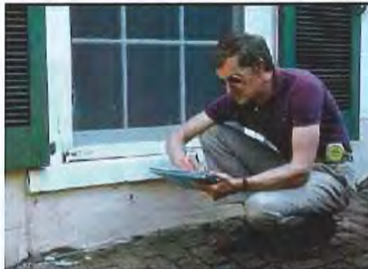
Window condition assessment preceding repair work.
