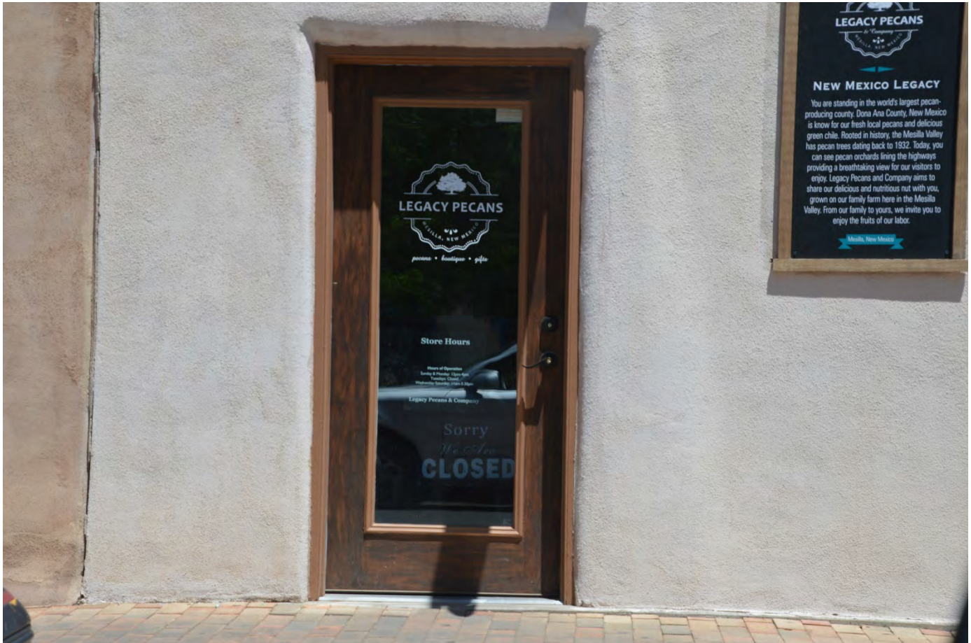
PHOTO OF DOOR AND DOOR JAMB TO BE REPAINTED
