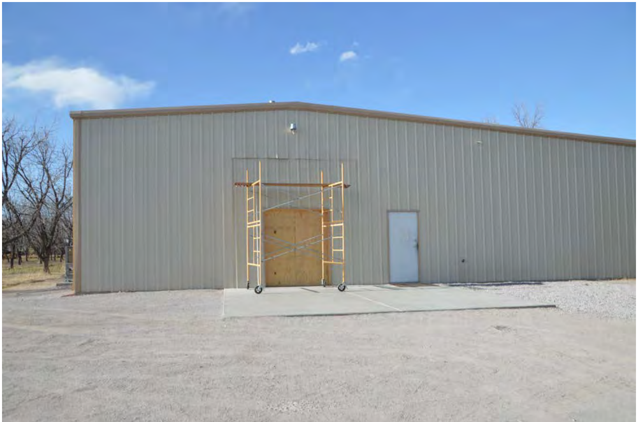
VIEW OF METAL BUILDING FROM UNIVERSITY AVENUE
