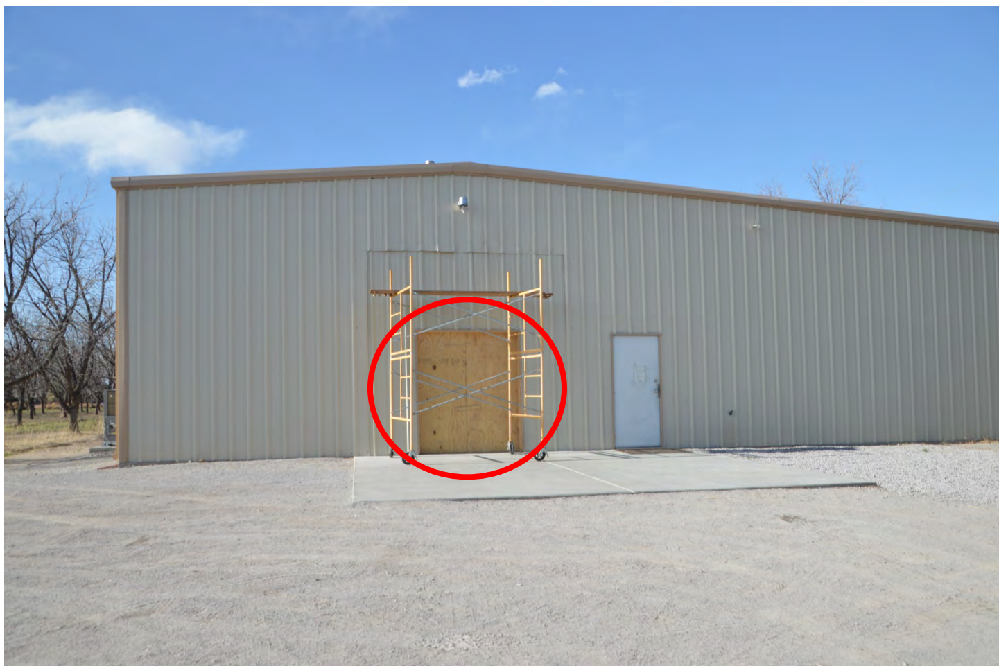
PHOTO OF METAL BUILDING SHOWING DOOR BEING REPLACED
