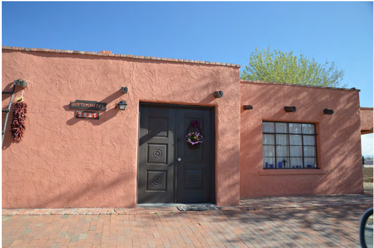
PHOTO OF FRONT OF DWELLING SHOWING ENTRYWAY
