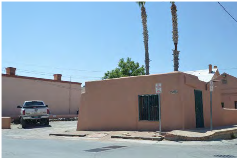
STRUCTURE FROM CALLE DE SANTIAGO
