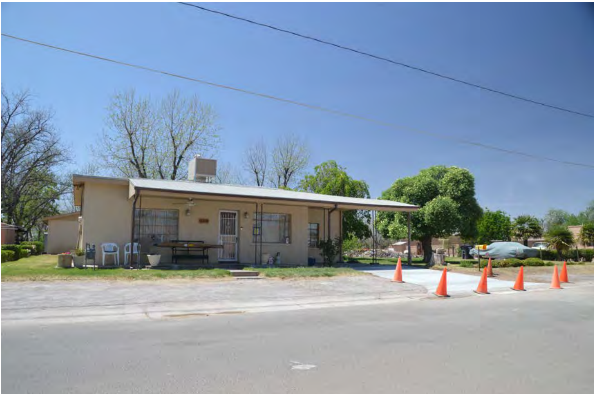
PHOTO OF SUBJECT STRUCTURE AND DRIVEWAY FROM CALLE PRINCIPAL
