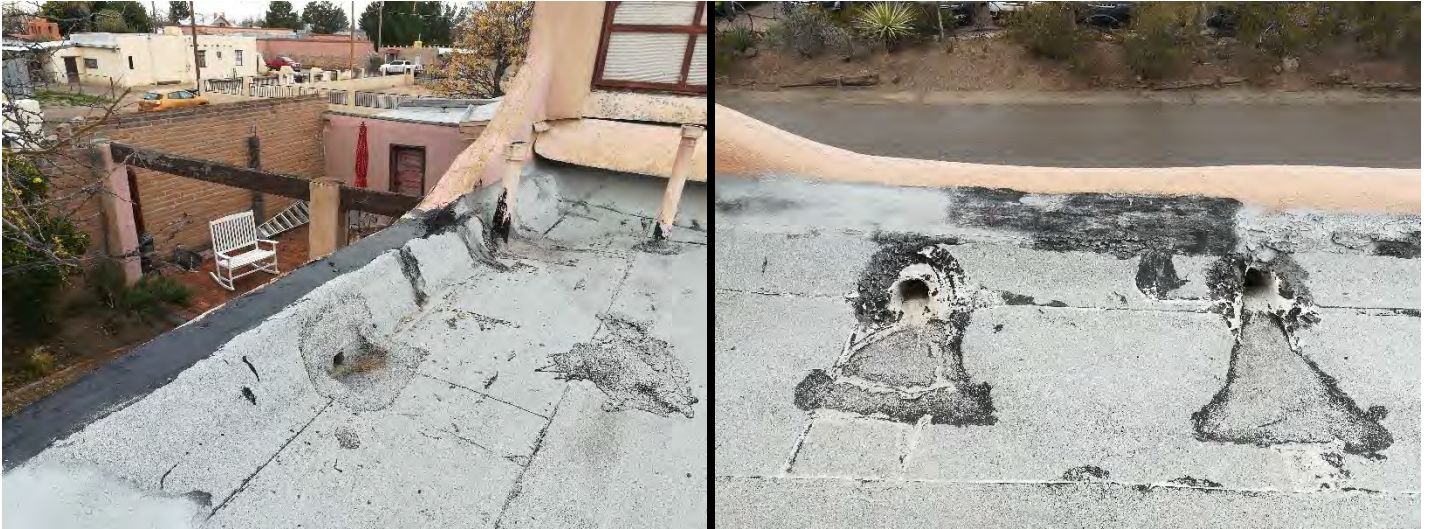
Photos: East roof section. Complete BUR removal and replacement.
