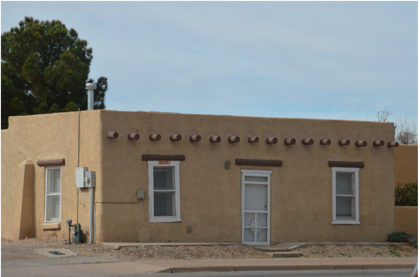
PHOTO OF NEARBY RESIDENTIAL RENTAL UNIT
