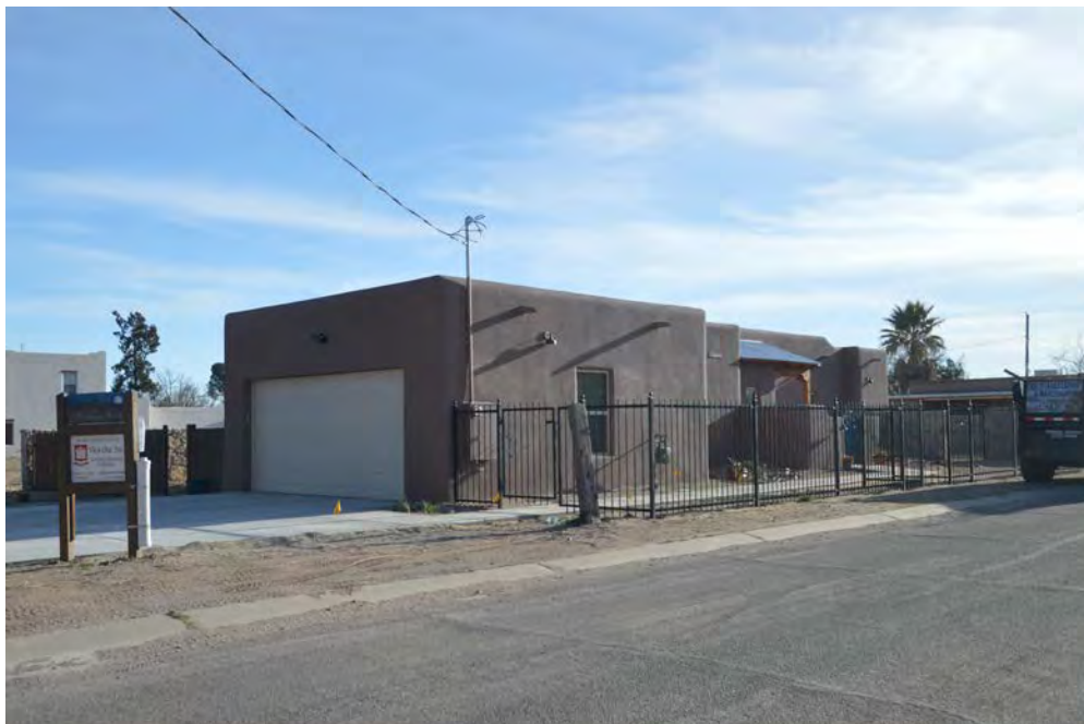
PHOTO OF DWELLING FROM CALLE DE COLON
