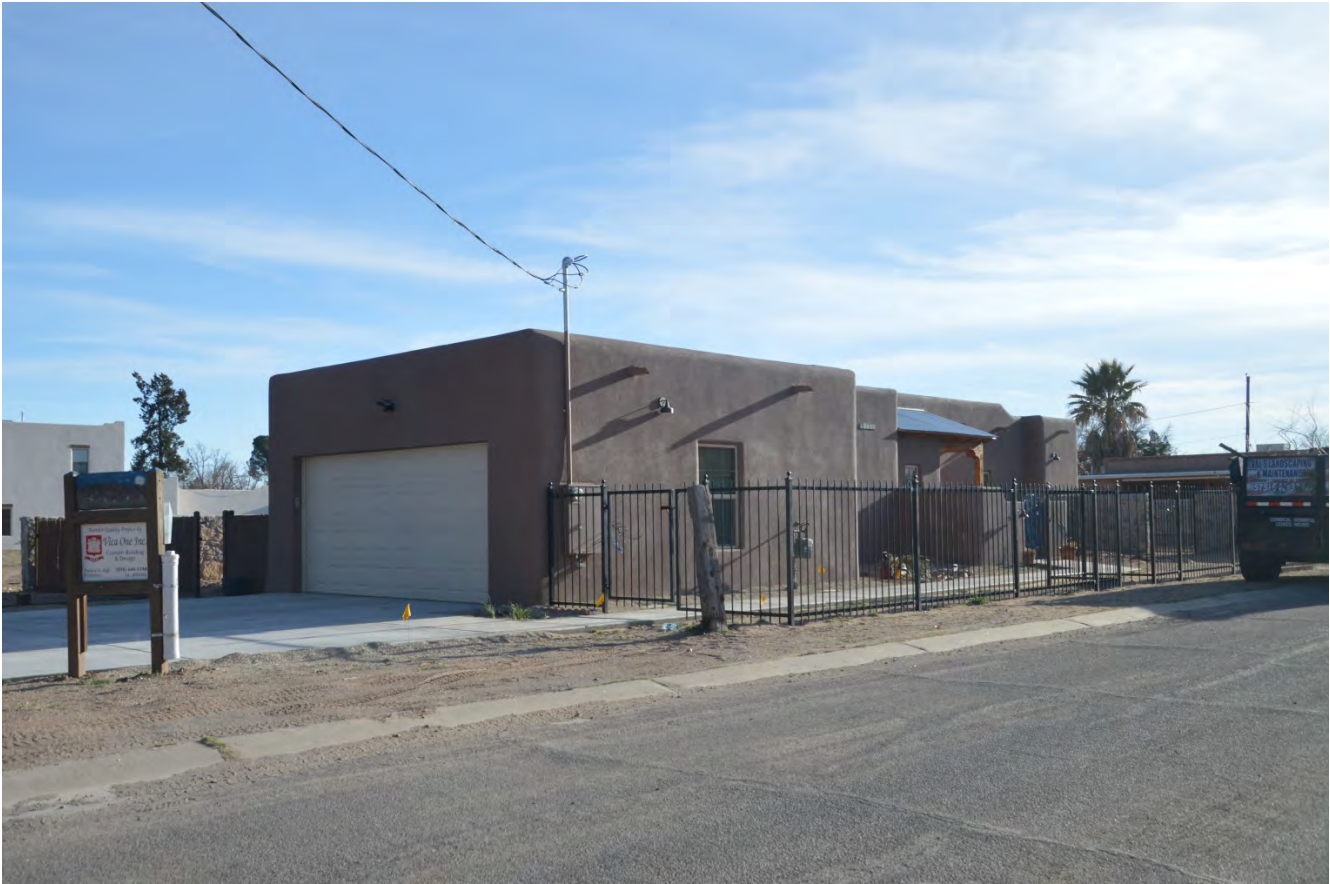
PHOTO OF THE RECENTLY BUILT DWELLING AT 2305 CALLE DE COLON
