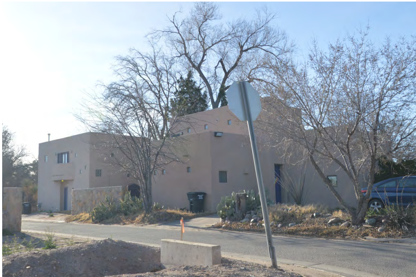
PHOTO OF THE TWO STORY DWELLINGS ACROSS CALLE DE COLON TO THE NORTH
