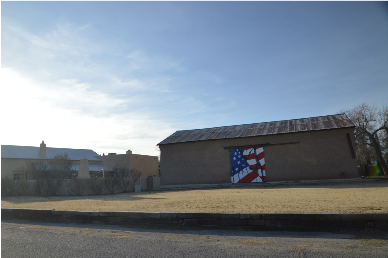
PHOTO OF THE LARGE DWELLING AND BARN AT 2350 CALLE DE PARIAN
