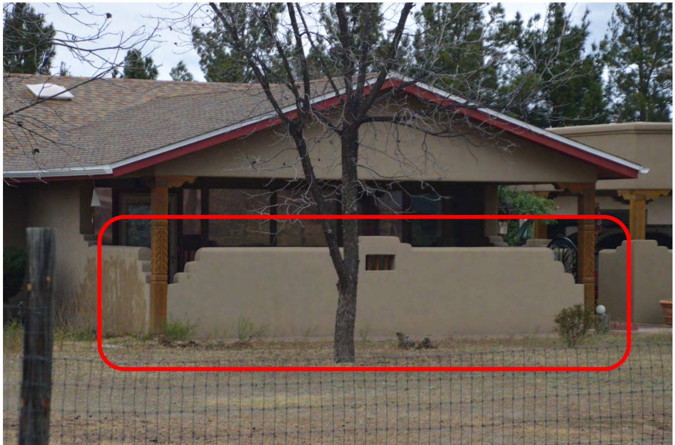
PHOTO SHOWING WALL AT FRONT OF HOUSE
