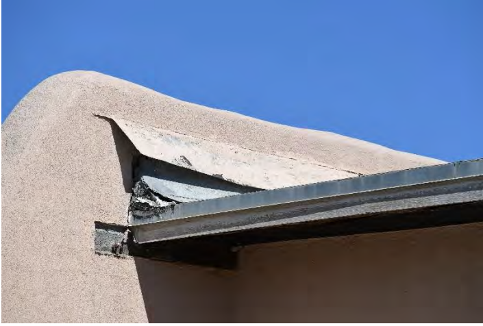
Photo: West roof section. All soffit and fascia will be removed and replaced
