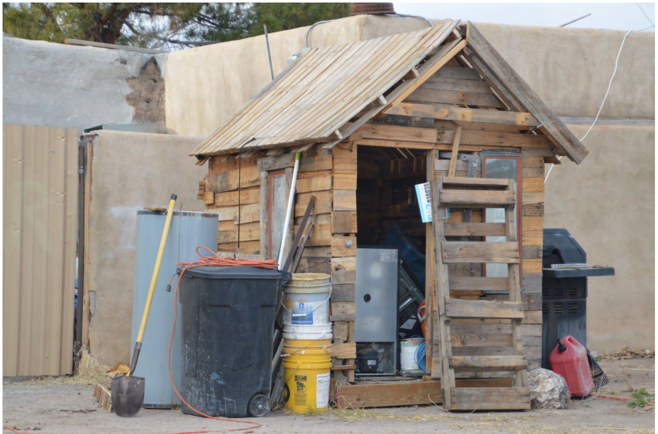
PHOTO OF SHED
