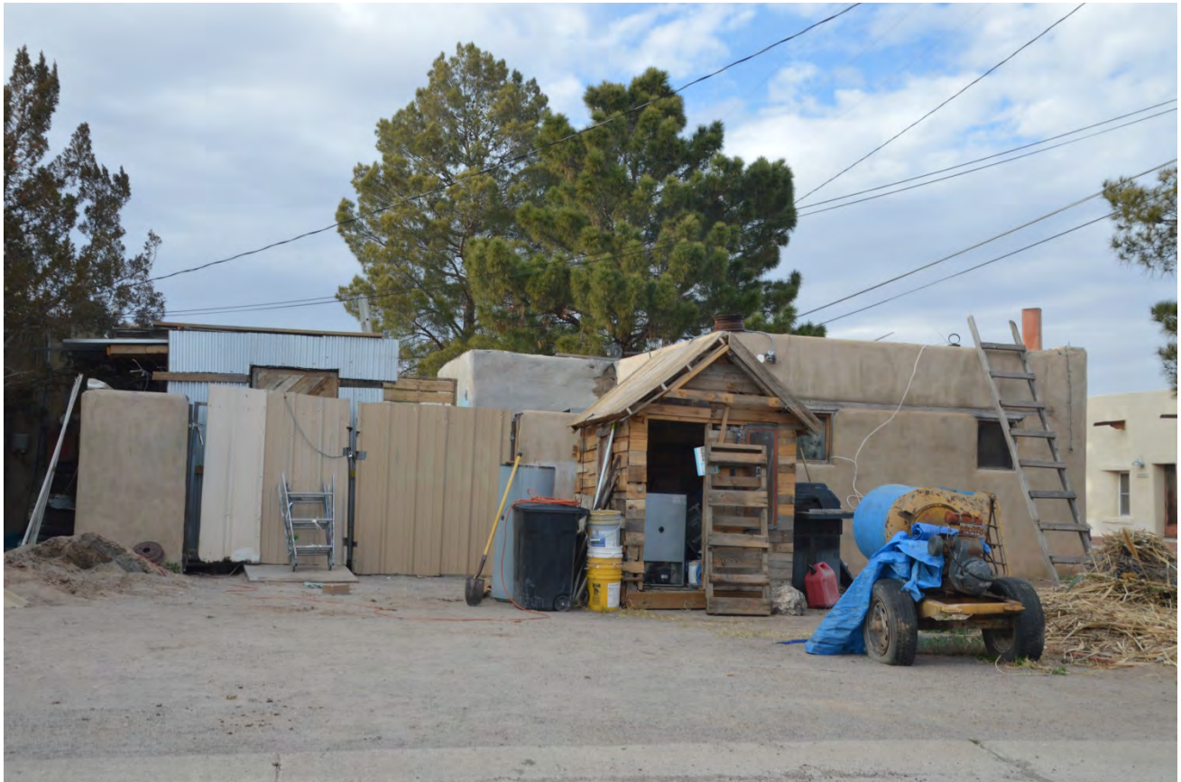
PHOTO OF SOUTH SIDE OF PROPERTY FROM CALLE DE COLON SHOWING SHED AND AREA TO BE FENCED
