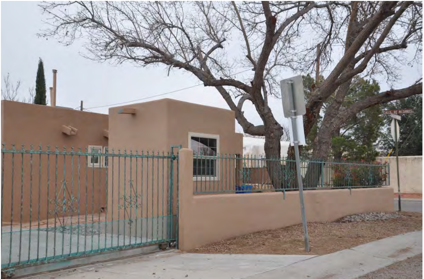
VIEW OF PROPERTY FROM CALLE DE PRINCIPAL
