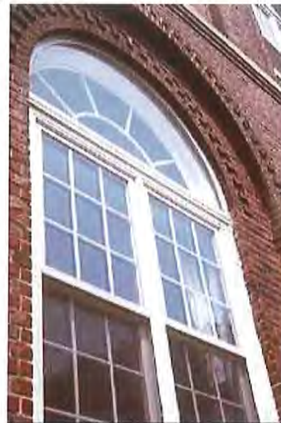
Newly painted double-hung wood windows.
