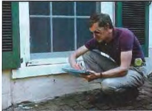
Window condition assessment preceding repair work.
