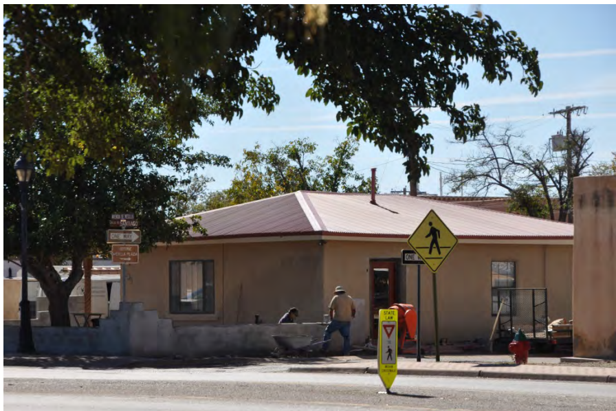
STRUCTURE FROM AVENIDA DE MESILLA
