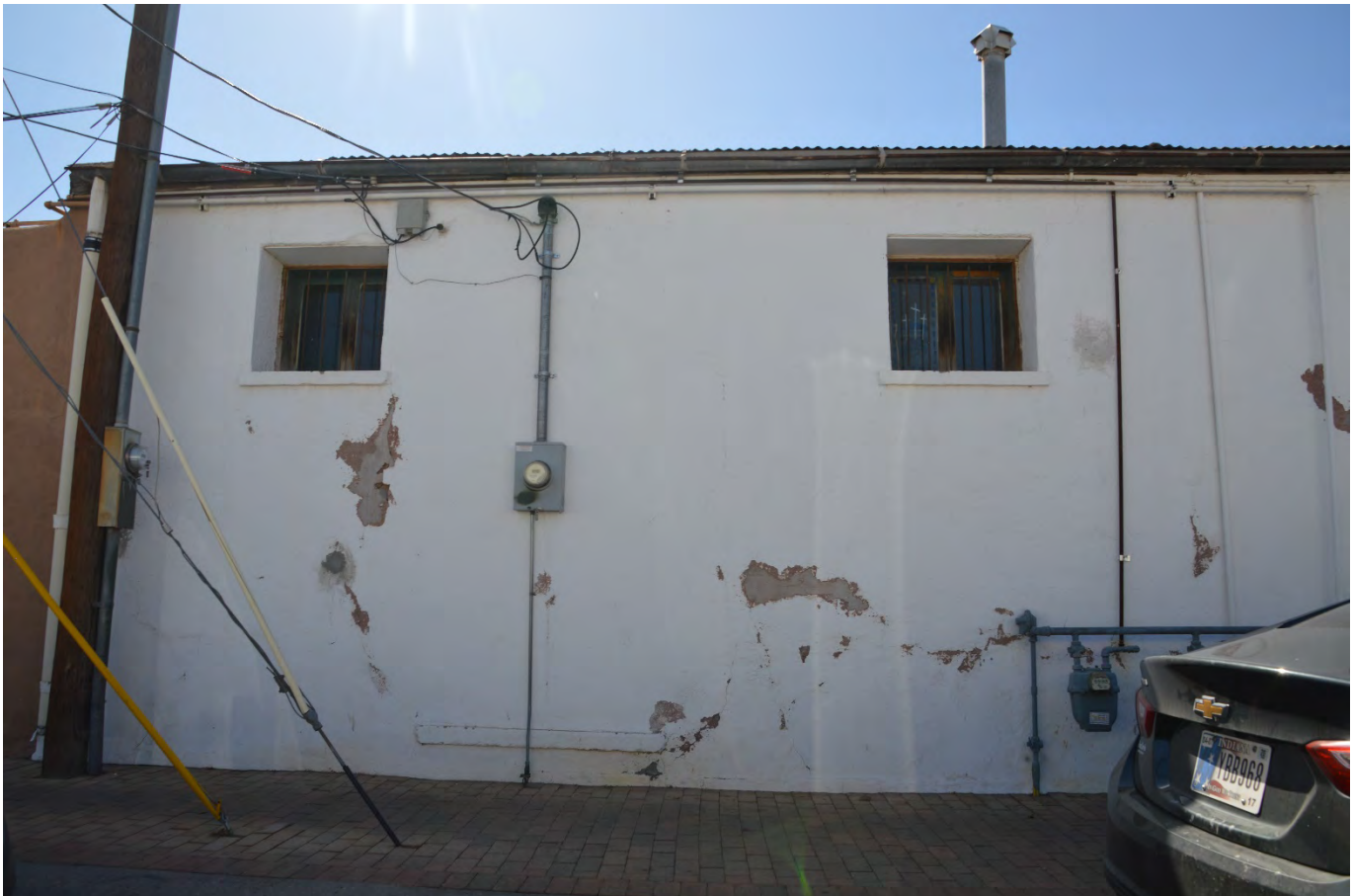
PHOTO OF THE STRUCTURE FROM CALLE DE GUADALUPE
