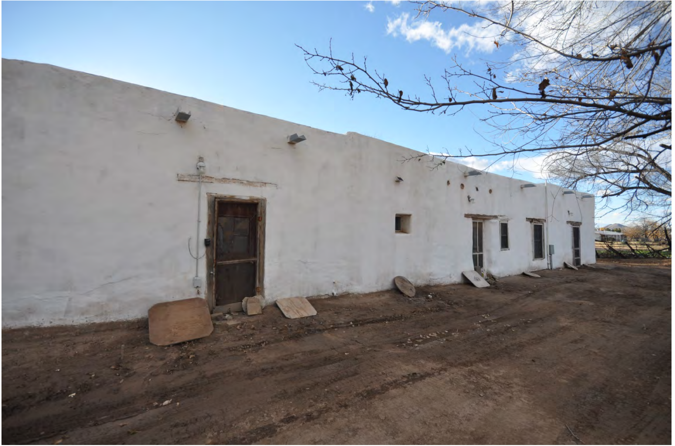
PHOTO OF THE REAR OF THE DWELLING
