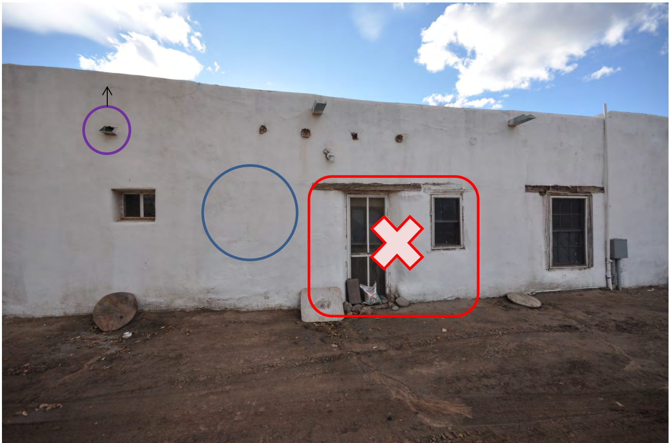
PHOTO OF THE REAR OF THE DWELLING SHOWING THE DOOR AND WINDOW TO BE CLOSED, THE PROPOSED LOCATION OF THE WINDOW BEING MOVED FROM THE FRONT, AND THE CANALE TO BE RELOCATED HIGHER
