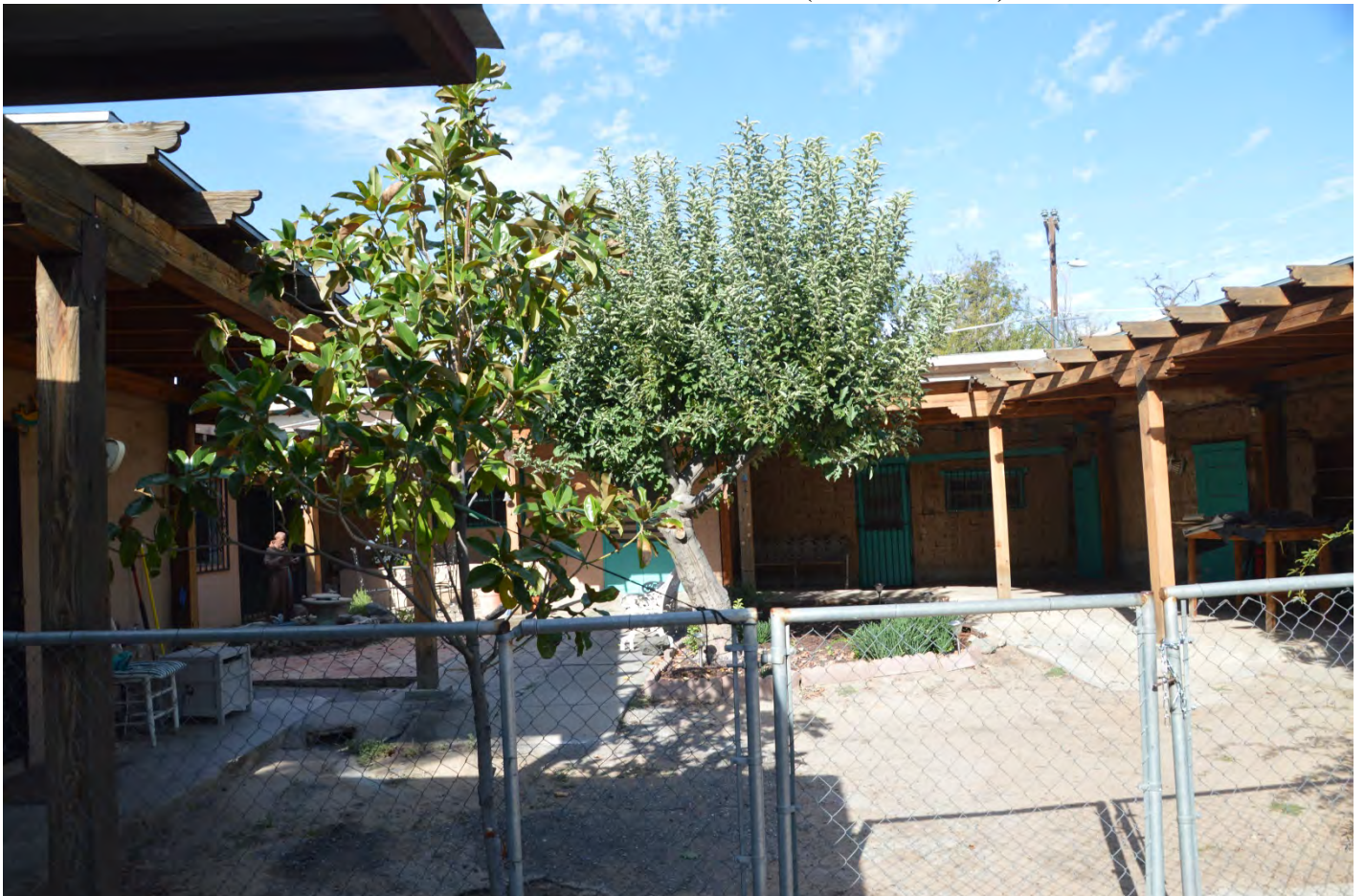
PHOTO OF REAR OF DWELLING (Taken 10/19/17)
