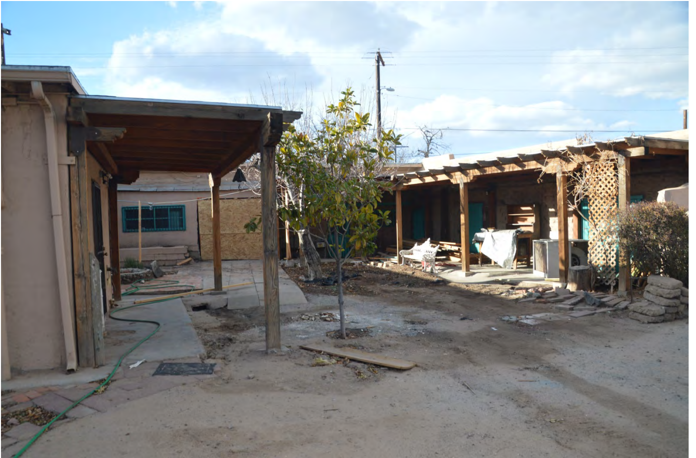
PHOTO OF REAR OF DWELLING (Taken 12/27/18)
