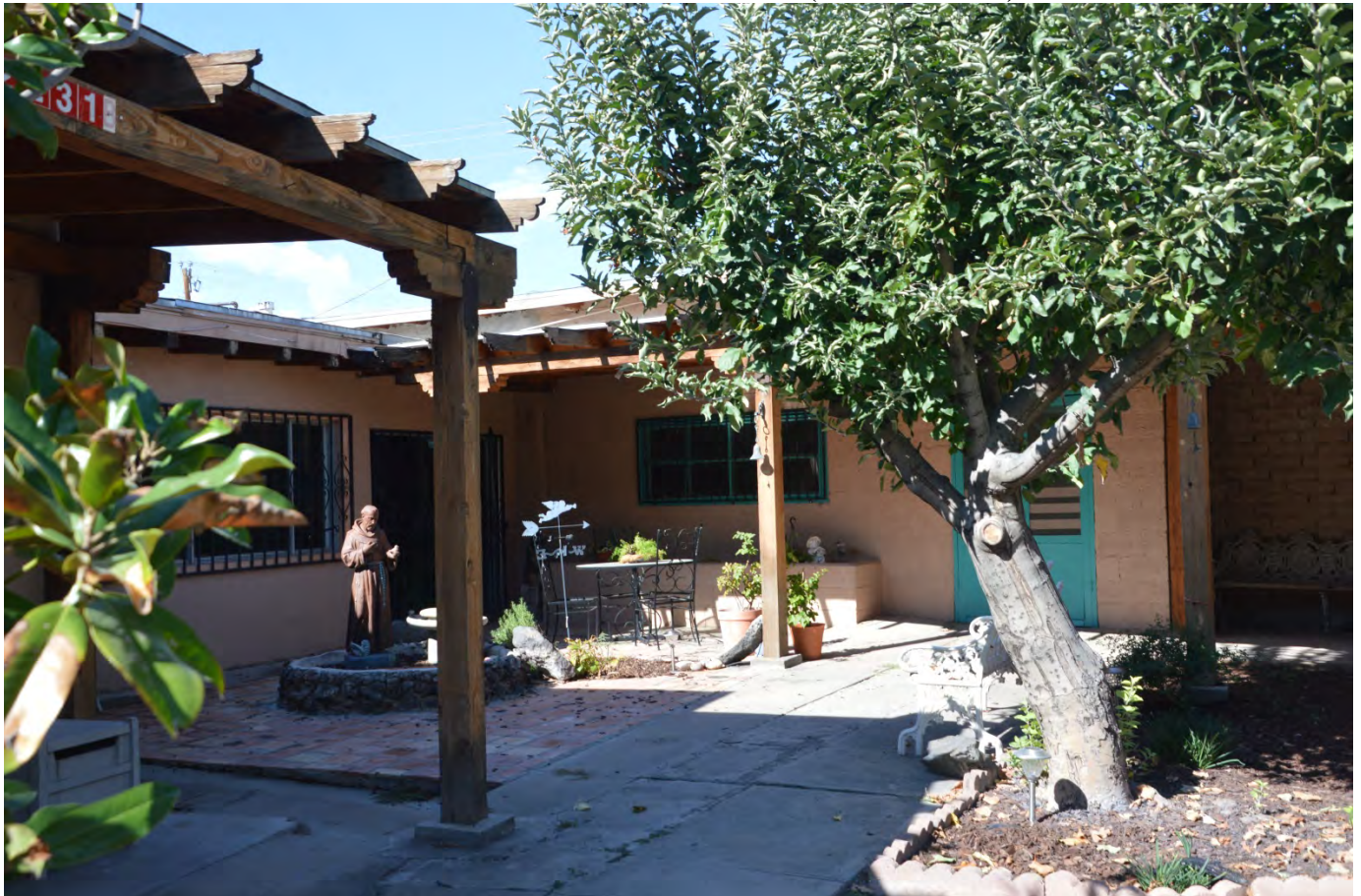
PHOTO OF REAR OF DWELLING (Taken 10/19/17)
