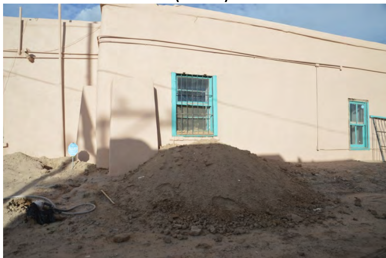
PHOTO OF REAR OF DWELLING SHOWING DIRT (ADOBE) REMOVED FROM INTERIOR (Taken 12/27/18)
