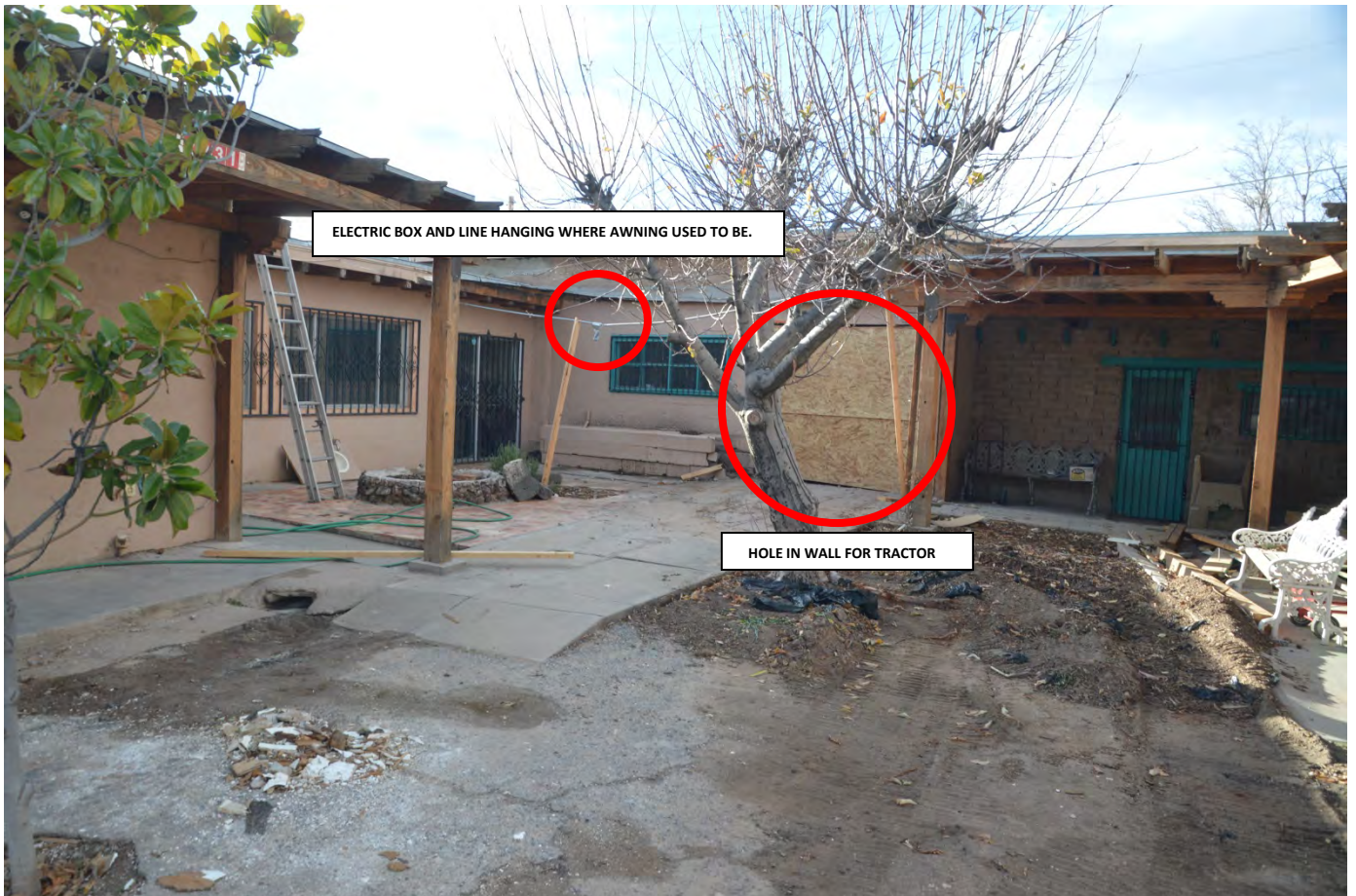
PHOTO OF REAR OF DWELLING (Taken 12/27/18)
